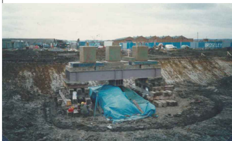
Plate load test (Load Test 2) ⑥
