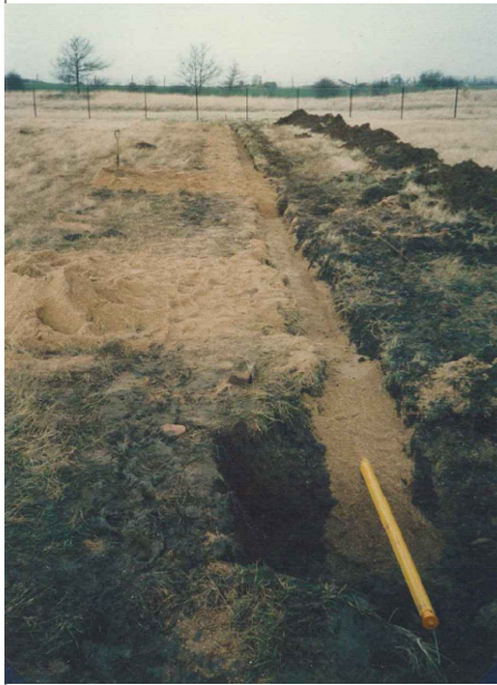
Horizontal inclinometer installed below earth fill ①
