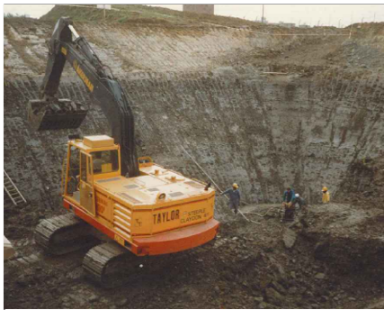
Excavation of load test area ②
