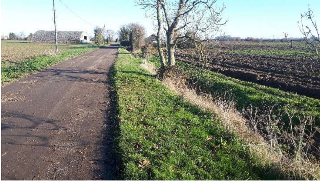
Plate 1 : Existing Land Drainage Ditch/Ordinary Watercourse (View east on from Perimeter Road)
