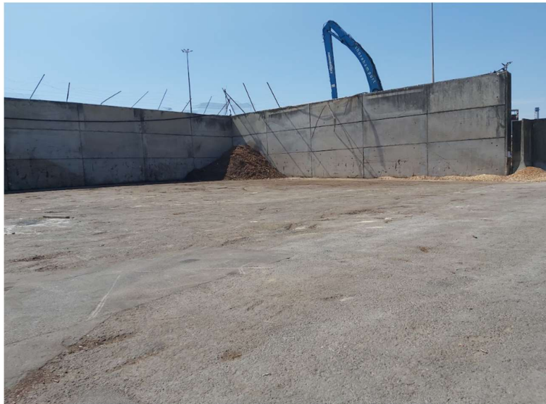
Figure 1 – Existing Concrete Bay Wall
