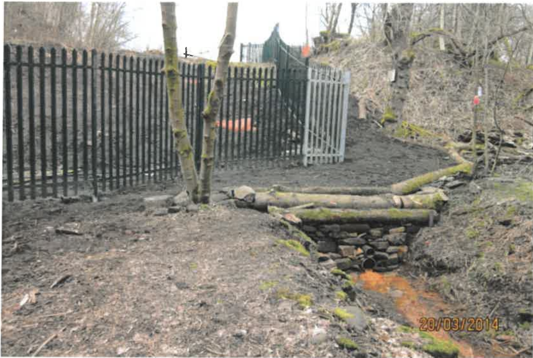
Picture 3: New headwall with realigned footpath and fencing.
