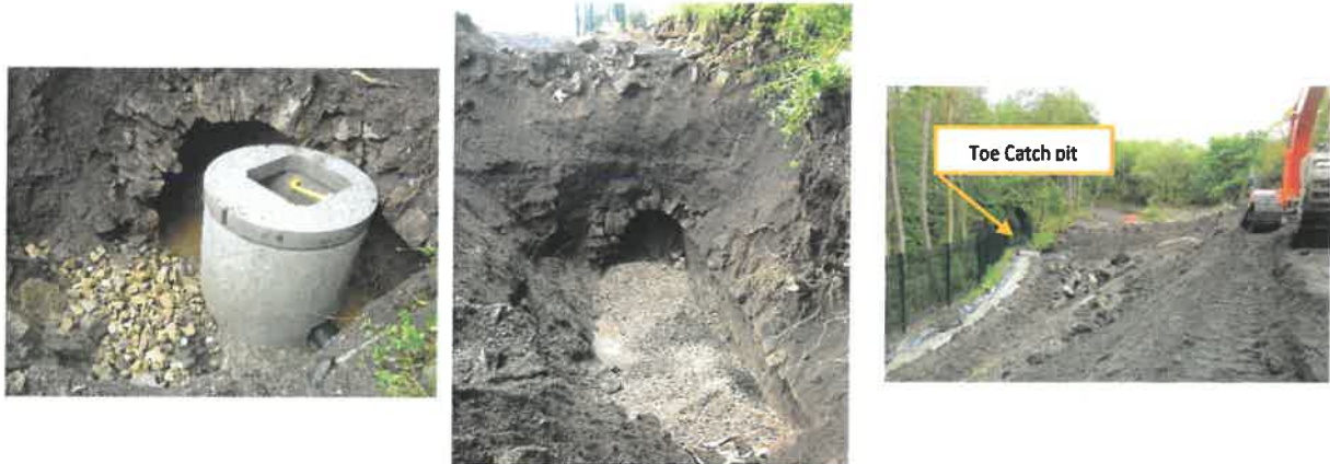
Fig 2.1.5 'Ochre' culvert Catch-pit ...with Replacement Pipe .....and Toe of Batter drain.
