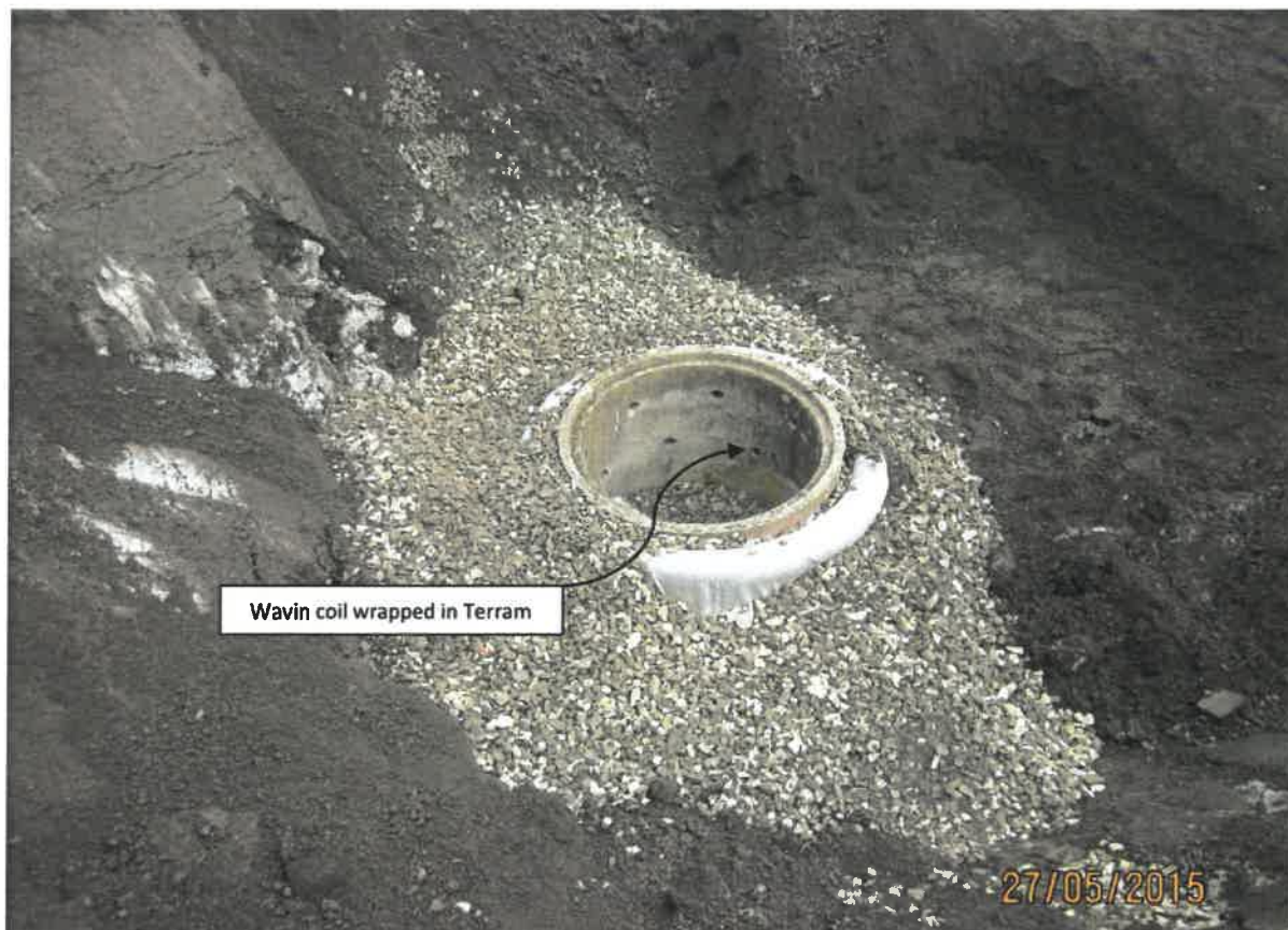
Figure 2.1.1 – Lower section of the new leachate chamber.
