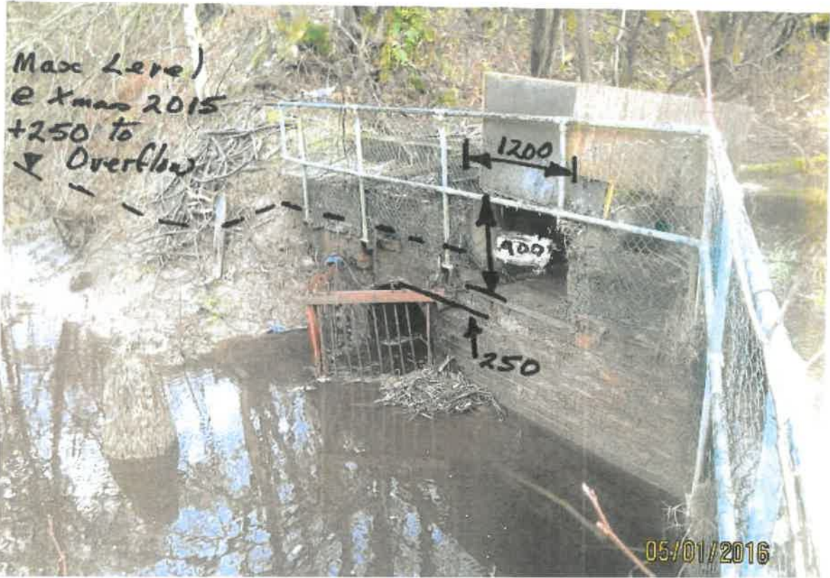
Figure 2.6.3 Existing lodge overflow arrangement.
