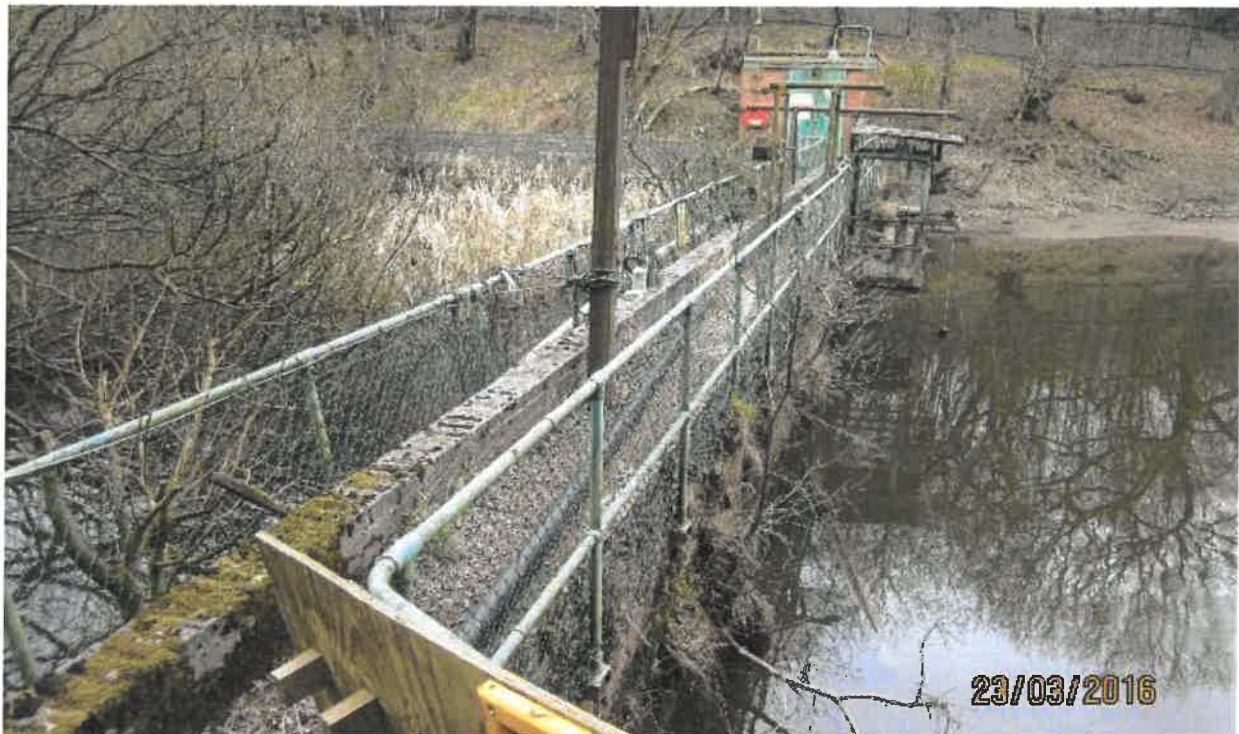
Figure 2.6.1 The concrete dam (the 'Old Tip' is located to the left).
