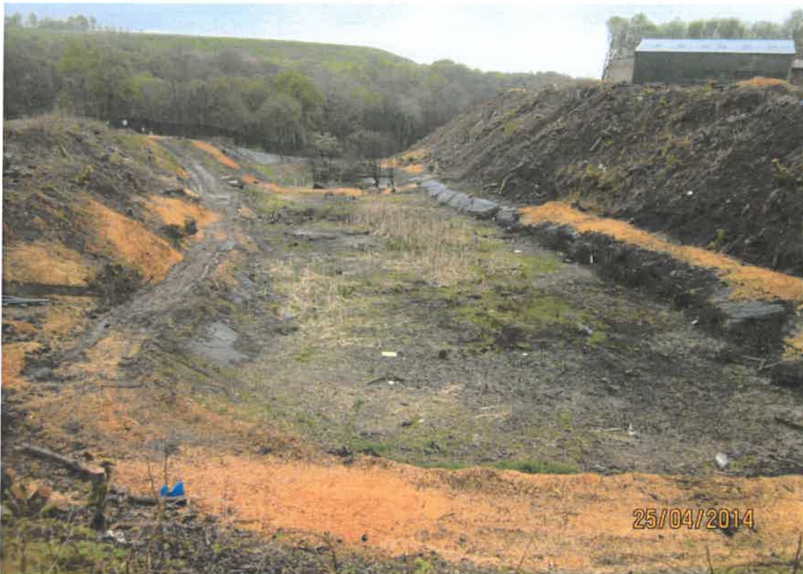
Picture 2: General work area looking east down the New Tip valley.
