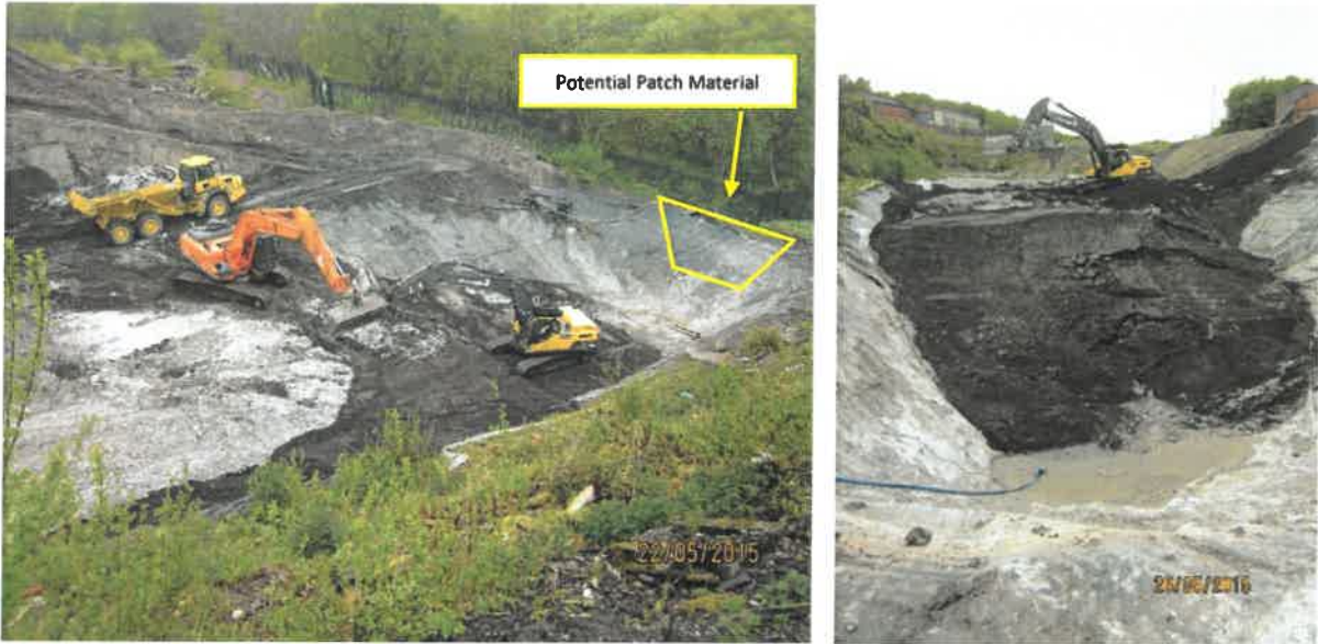
Figure 2.1.3 – Initial ash partition installation and paper pulp removal works.
