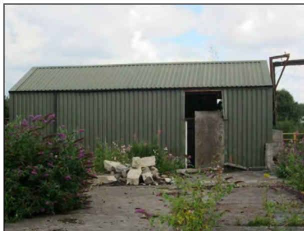
Photo 2: West elevation of Building E
