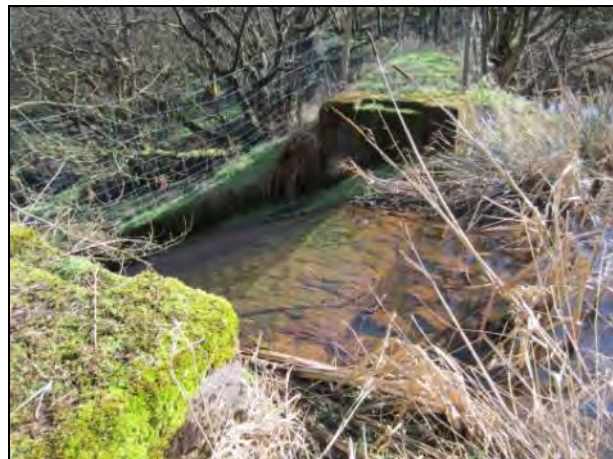
Photo 8: Concrete outfall from Pond 7
