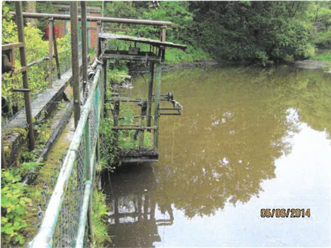
PHOTO 3 – VIEW OF SAMPLING PLATFORM AND VARIOUS FRAMES ALONG LENGTH OF DAM
