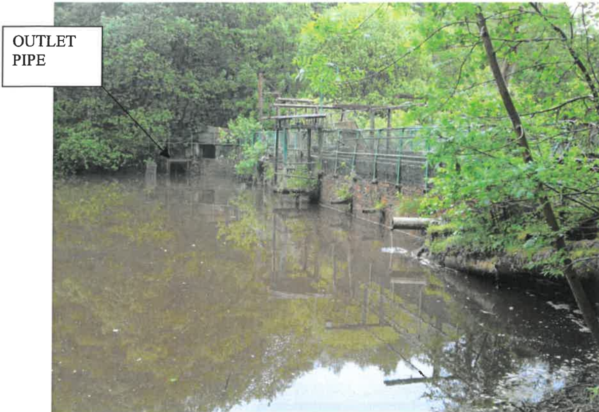
PHOTO 1 – VIEW OF DAM FROM SOUTH SIDE
