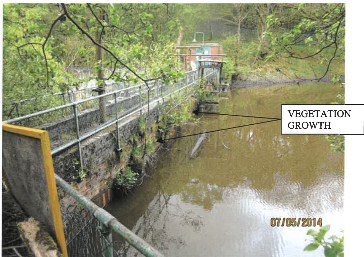
PHOTO 2 – VIEW OF DAM FROM NORTH SIDE
