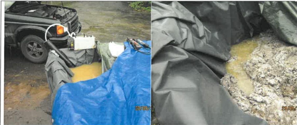
Skip 2 leachate sampling, 28/05/14
