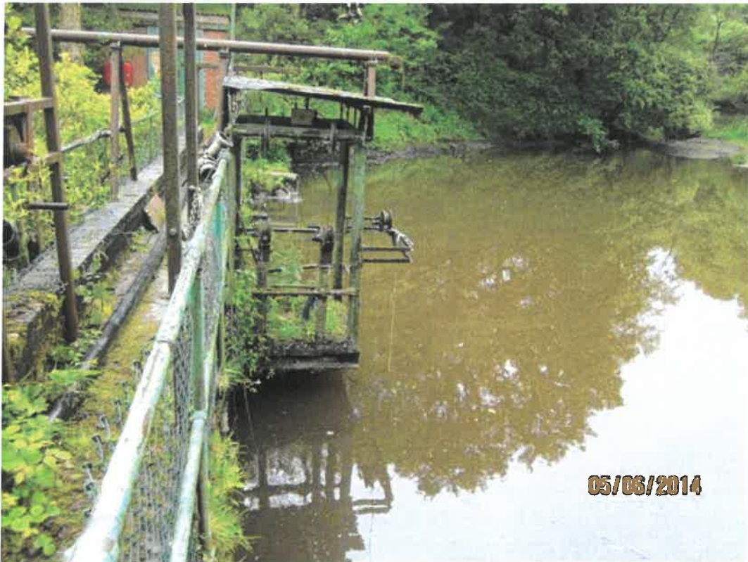
PHOTO 3 – VIE OF SAMPLING PLATFORM AND VARIOUS FRAMES ALONG LENGTH OF DAM
