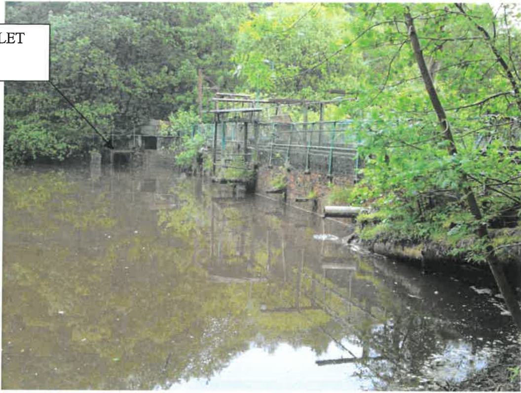
PHOTO 1 – VIEW OF DAM FROM SOUTH SIDE
