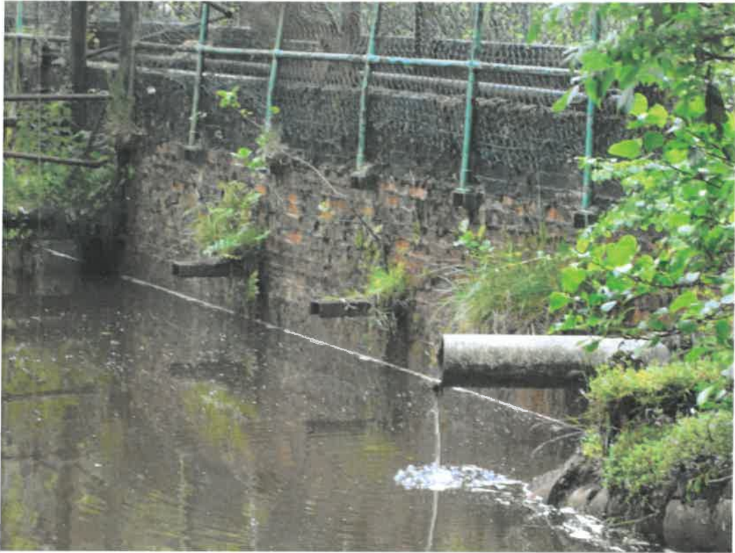
PHOTO 5 – VIEW OF SURFACE WATER INLET TO POND
