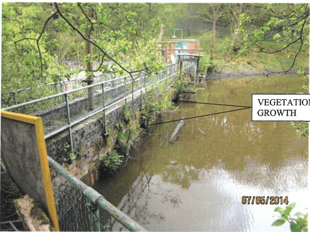
PHOTO 2 – VIEW OF DAM FROM NORTH SIDE
