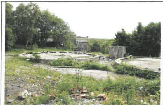
area of former fuel tanks in foreground; water tank bases to rear
