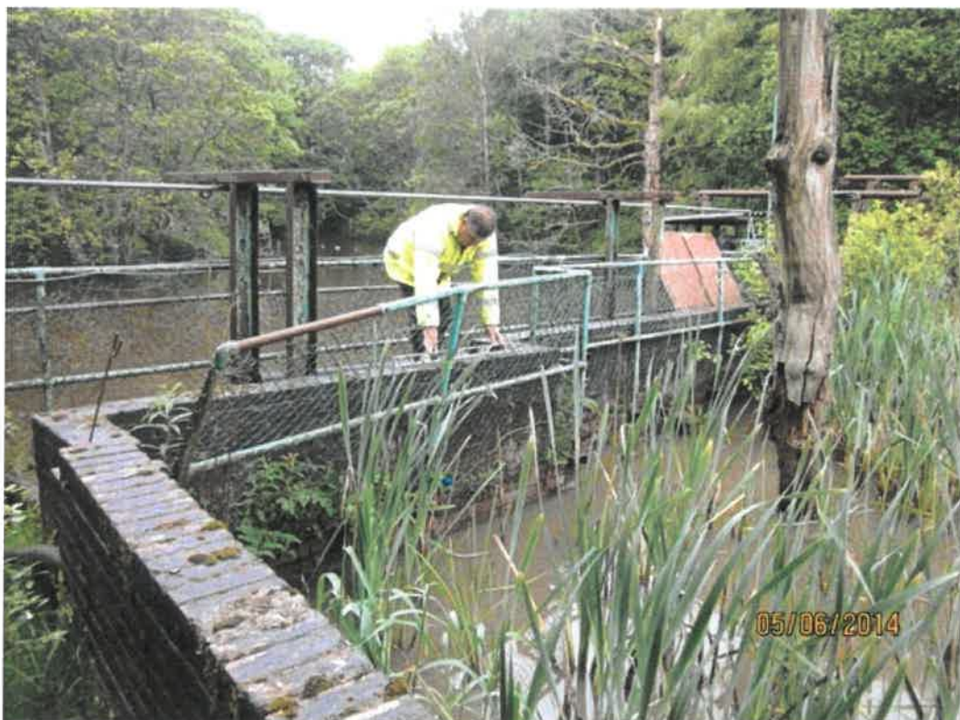
PHOTO 4 – VIEW OF FRONT FACE OF DAM
