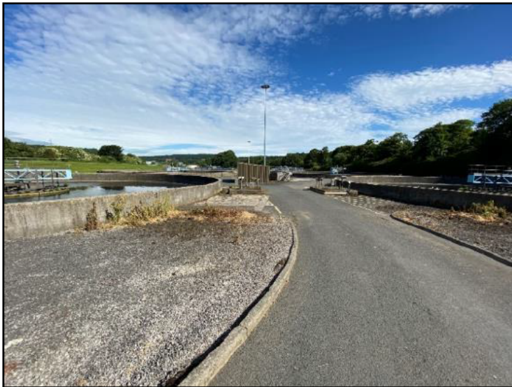
Figure 31 - Photo showing height of FST walls. There is no realistic pathway for sludge to enter these.
