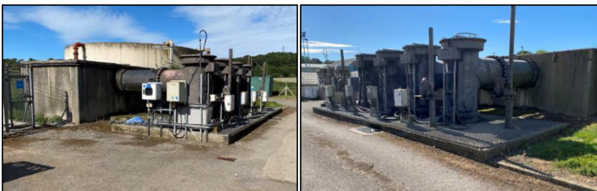
Figure 33. Final effluent chamber near the south conditioning feed tank in the DW area (west).
