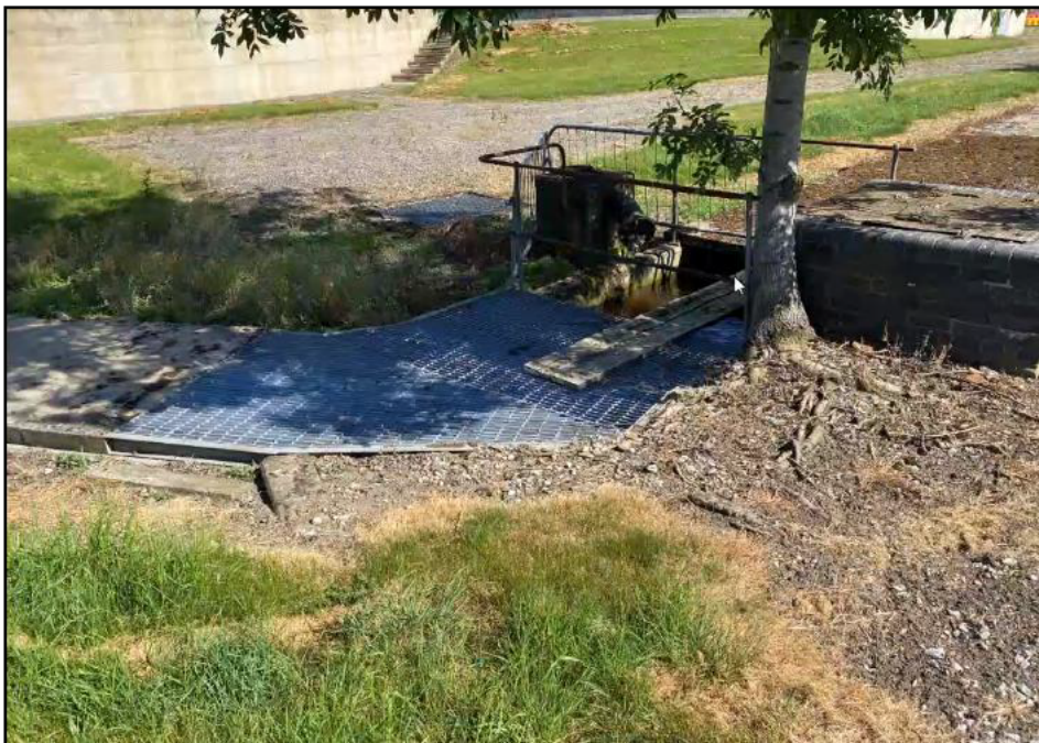
Figure 35. Sections of open decking on the channel feeding the humus tanks in the DW area (west).
