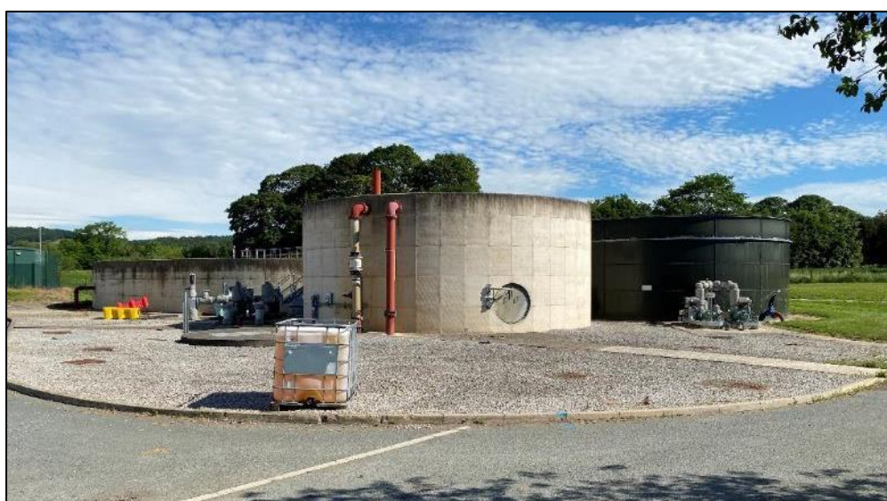
Figure 21. Centrate balance tanks.
