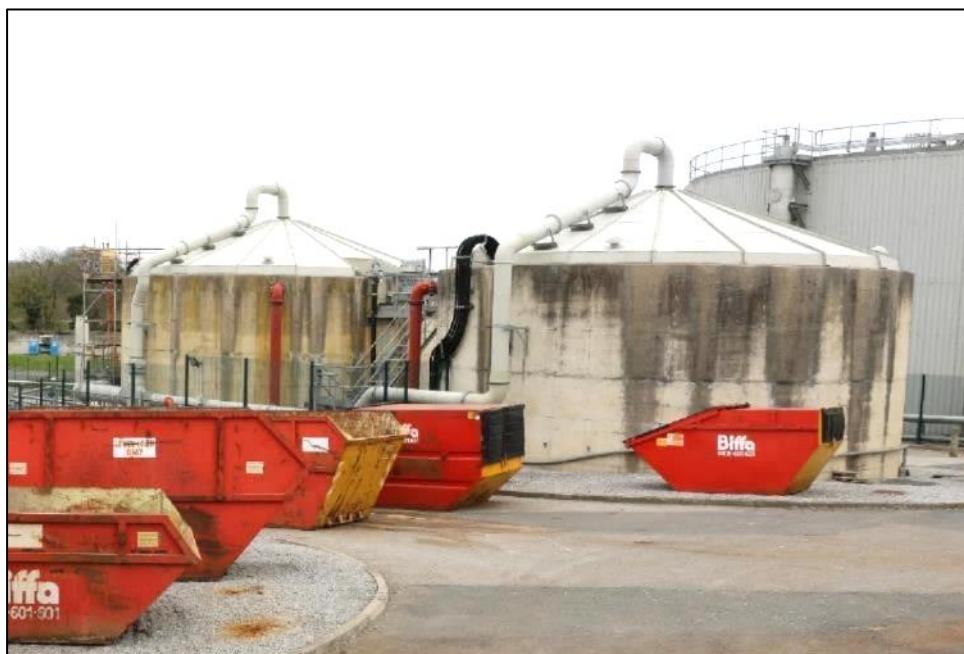
Figure 17. Degassing tanks.
