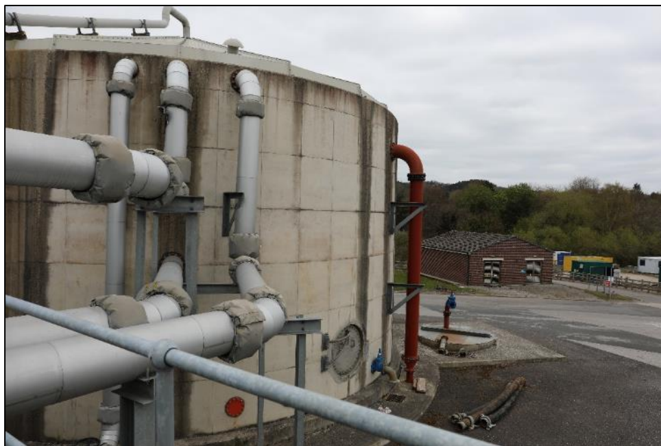
Figure 9. Sludge screen feed tank.
