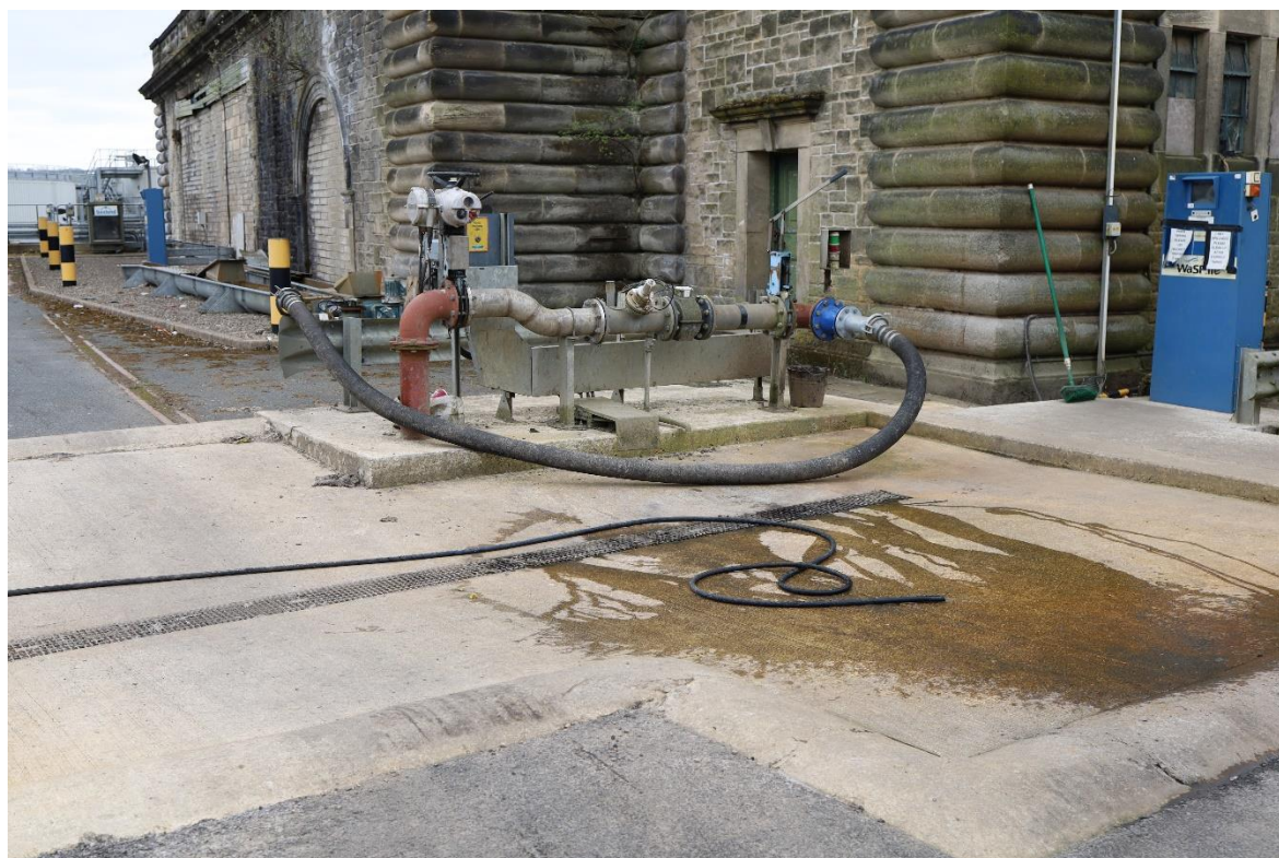
Figure D Sludge unloading area via WaSP loggers
