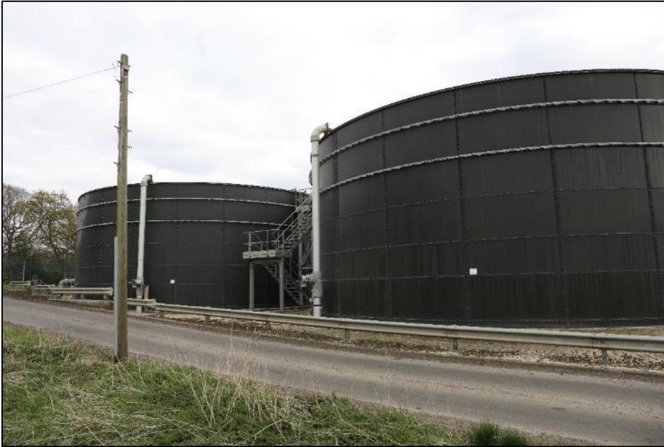
Figure 18. Export dewatering feed tanks.
