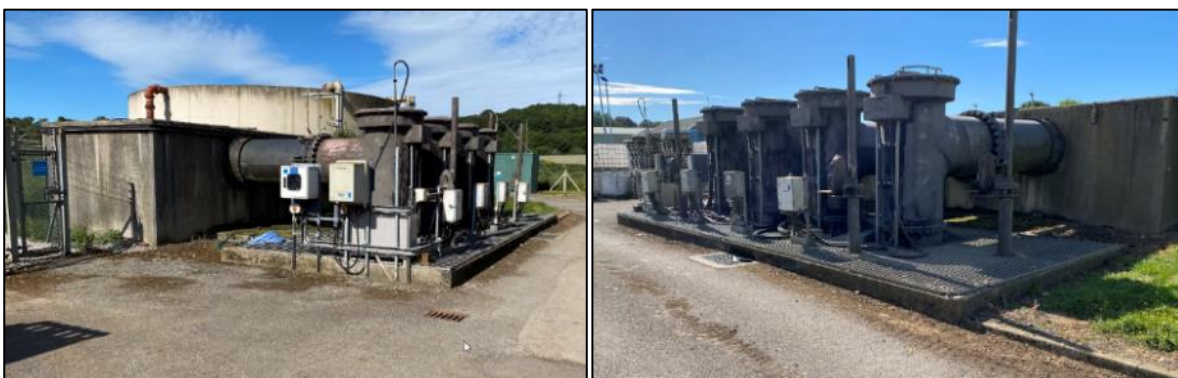
Figure 33. Final effluent chamber near the south conditioning feed tank in the DW area (west).
