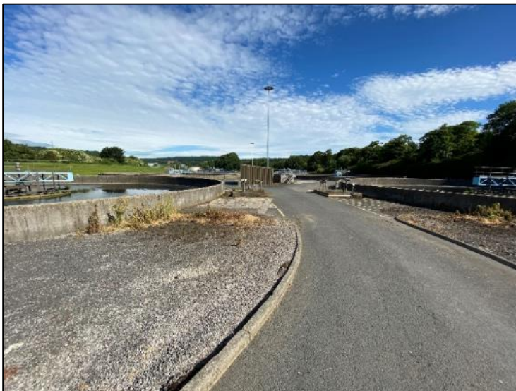
Figure 31 - Photo showing height of FST walls. There is no realistic pathway for sludge to enter these.
