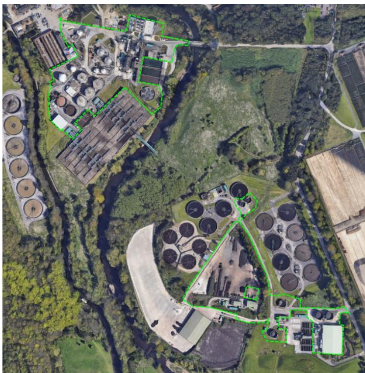
Figure 1. Esholt STF aerial view. Permit boundary in green. © Google, 2021
