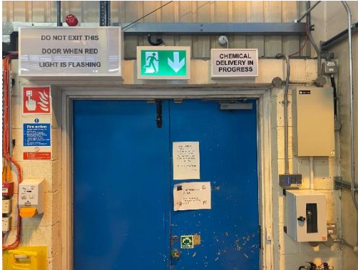
Delivery in progress sign and red beacon
