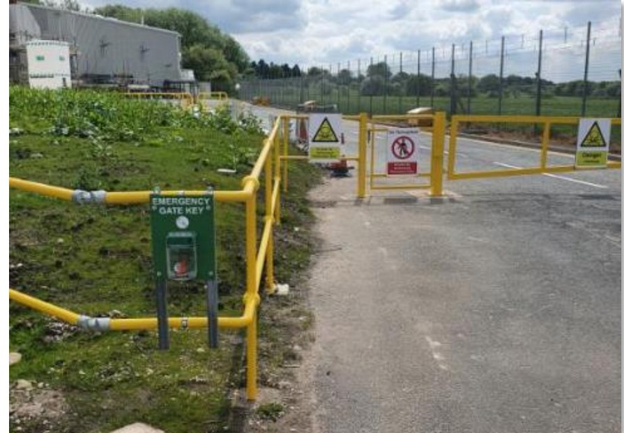
Figure 4: Gated entrance to new tanker unloading bay
