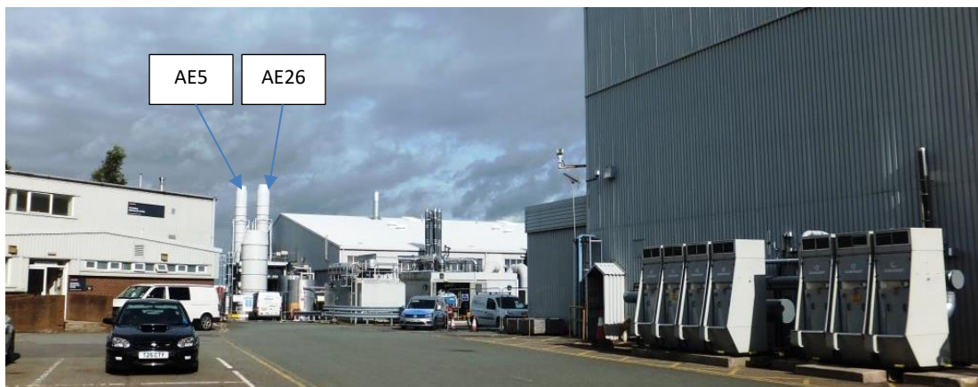
Photograph 11-1: View along southern edge of 3B (Machine Shop) towards scrubbers
