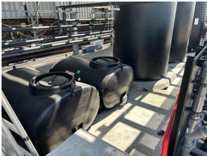
Photograph 3-1: View of bund showing gravity feed tanks T1007 and T1008
