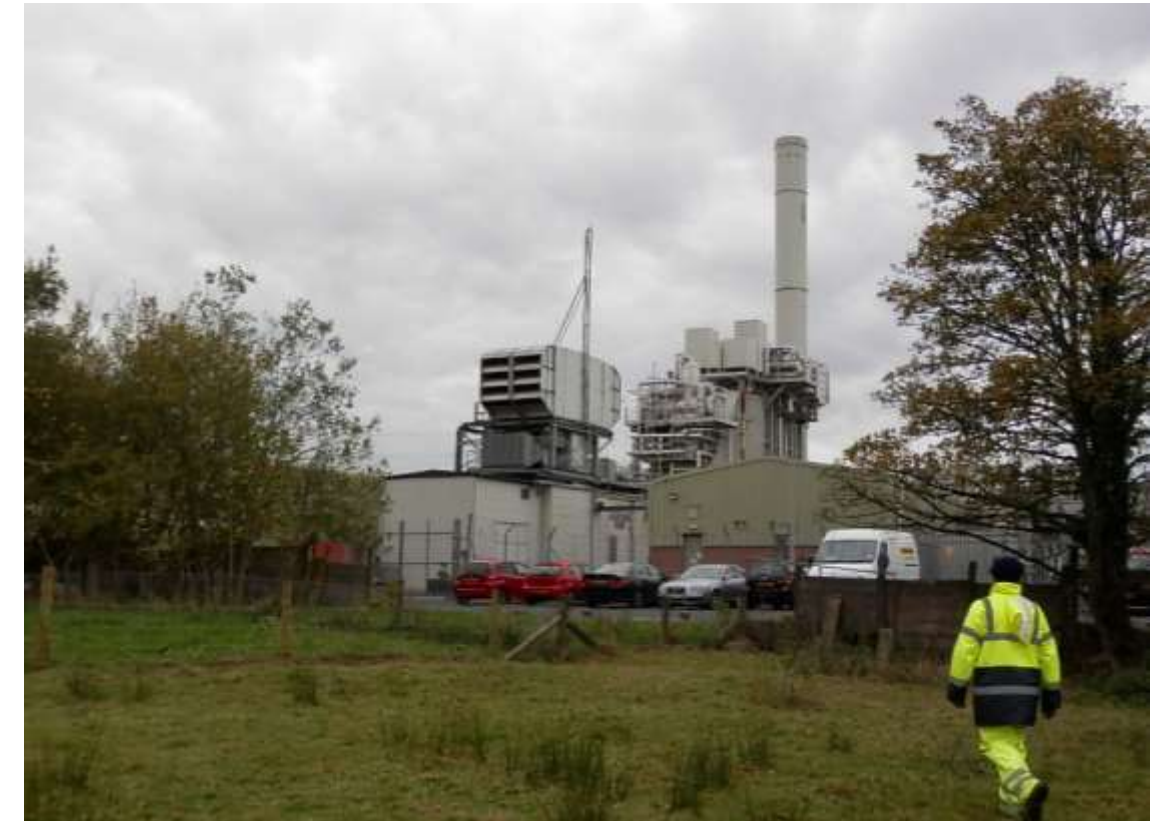
fig 19: view of the CHP plant from the north
