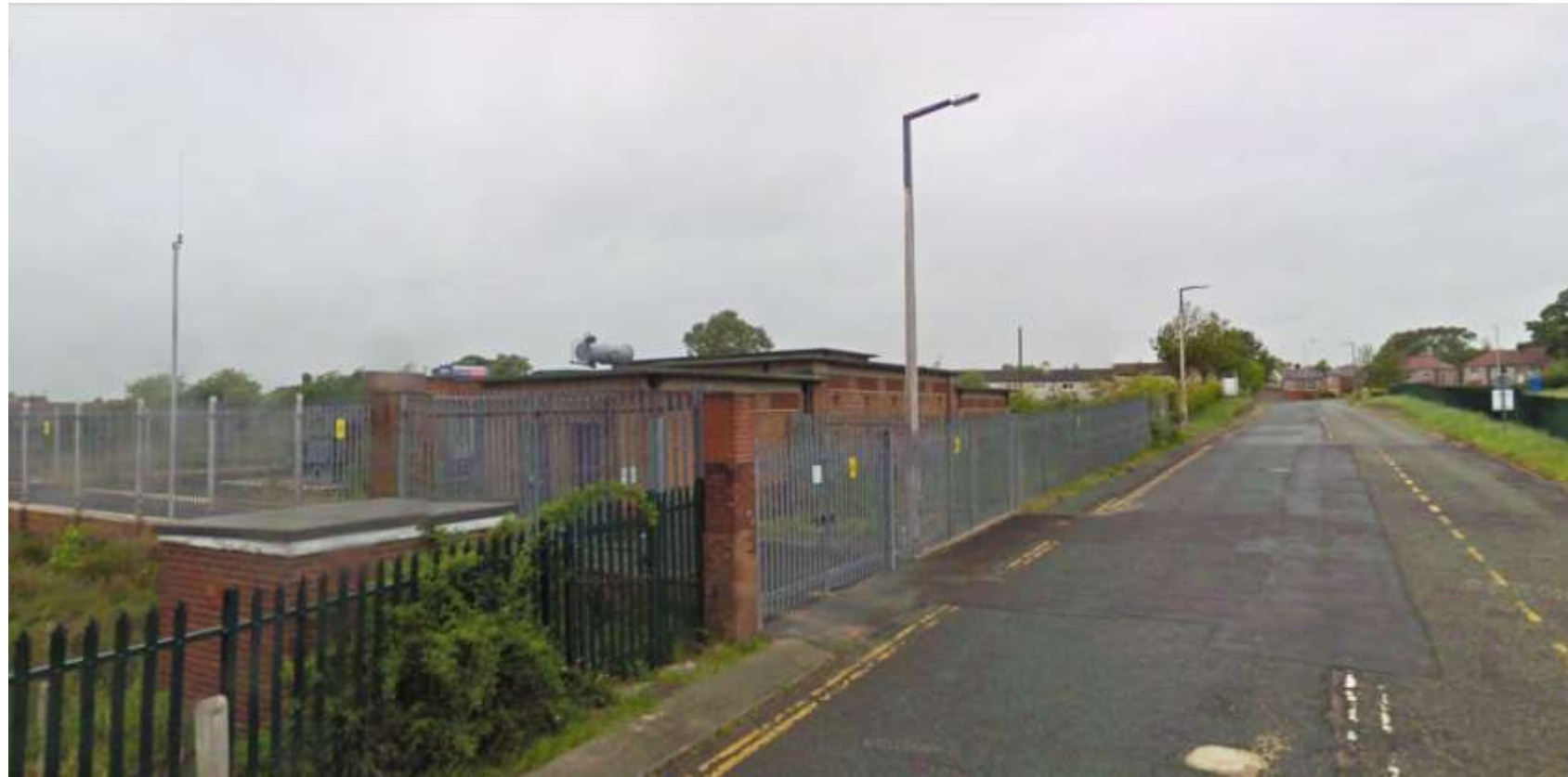
fig 4: view north past the substation to the Livesey Branch Road main entrance
