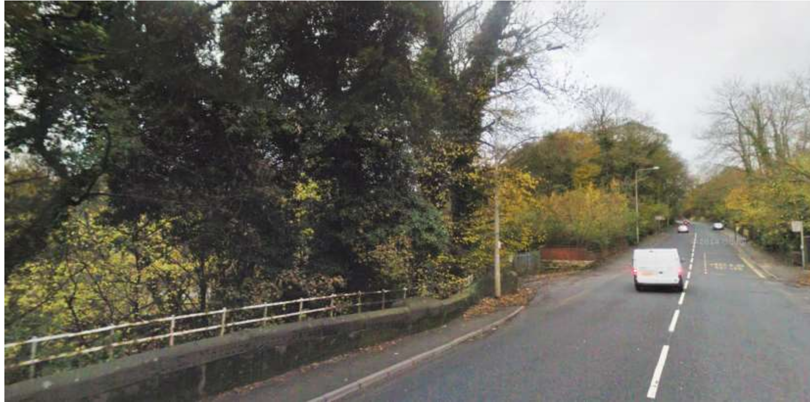
fig 13: Moulden Brow access on the left as seen from the east
