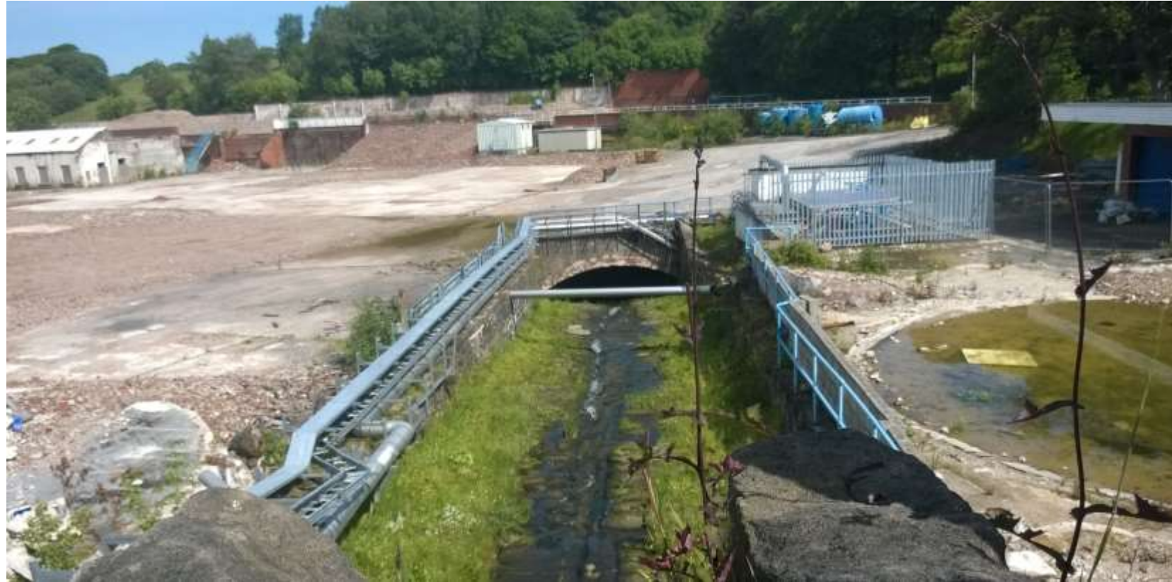
fig 28: the start of the culverted section of the River Roddlesworth
