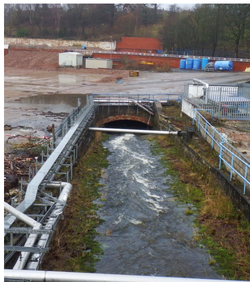
Figure 3.1: Culvert before surcharging
