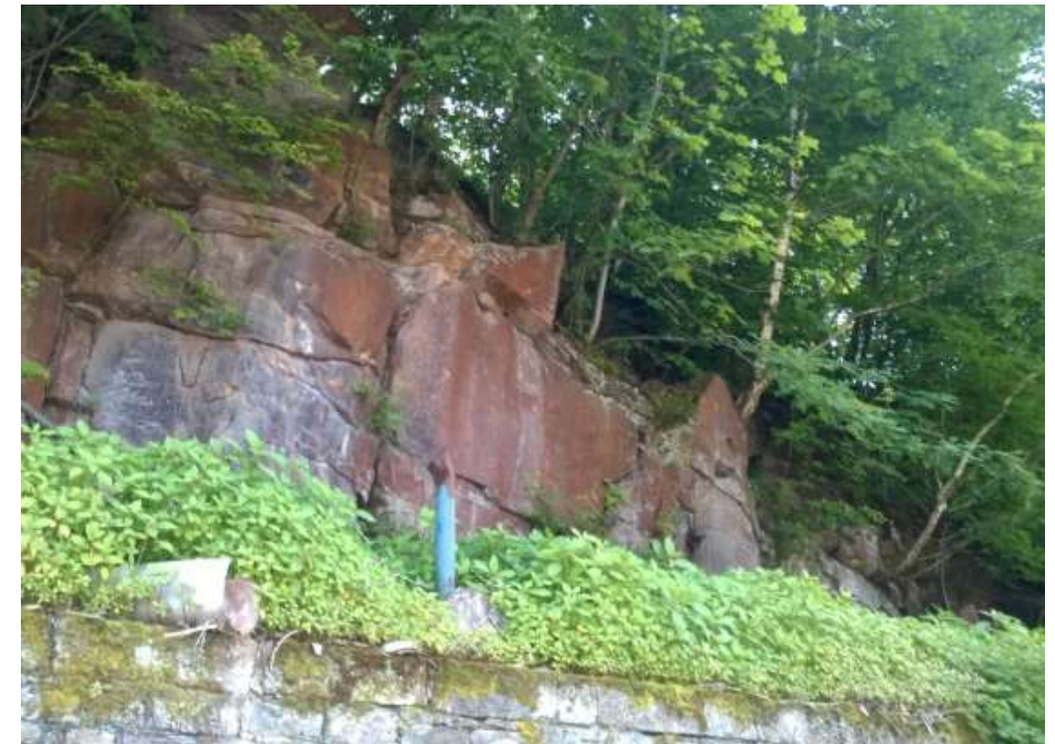
fig 31: steep sides and rock faces along the southern embankment
