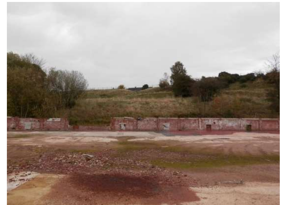
fig 7: view north across the valley floor toward the embankment
