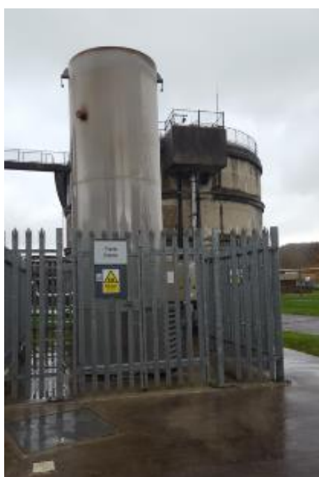
Photo 22: Biogas Flare
