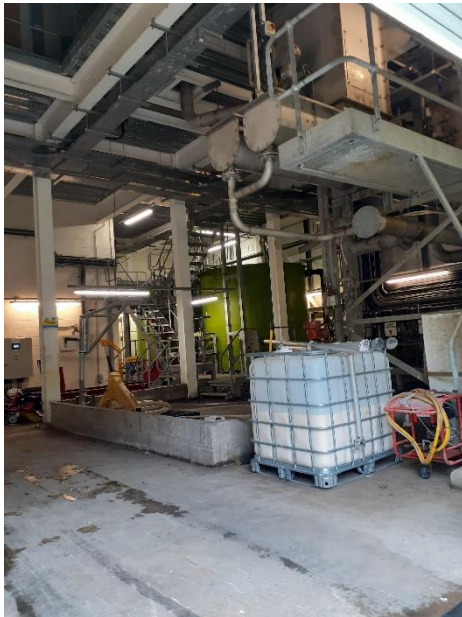
Photo 18: Dewatering Centrifuge Building
