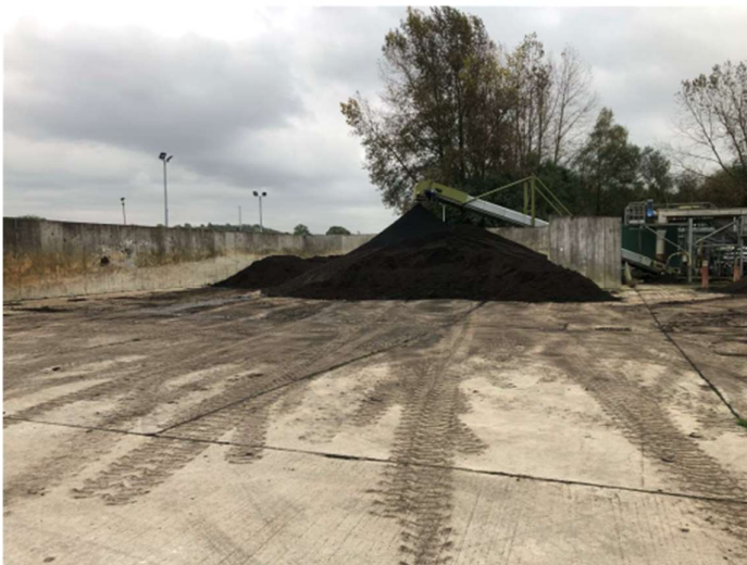
Photo 1: Digestate cake storage bay
