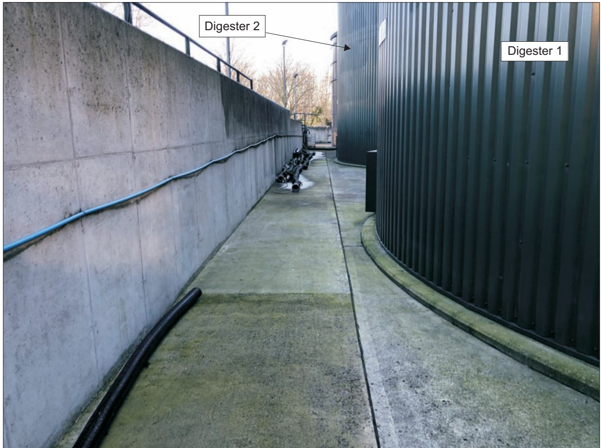
Photo 3. Base of secondary containment area along northern margin of digester tanks
