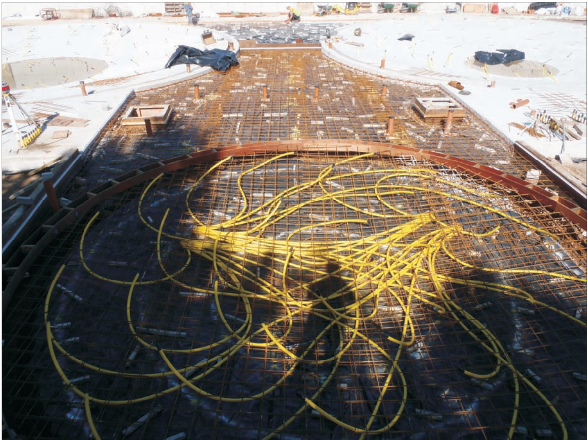
Photo 2. Buffer Tank base (during construction)
