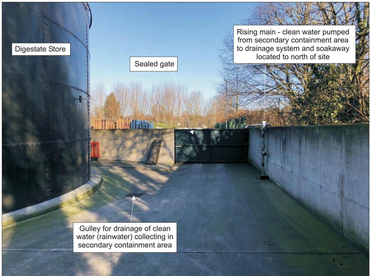
Photo 9. Retaining bund (walls) and sealed gate at north-eastern corner of site
