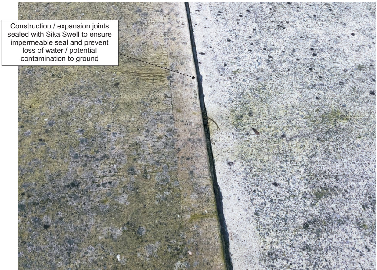
Photo 4. View of construction joint on base of secondary containment area
