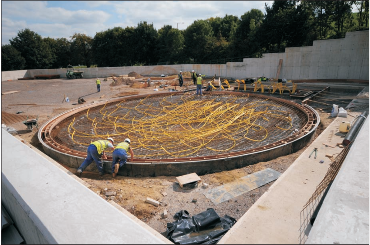
Photo 1. Digester 1 base (during construction)
