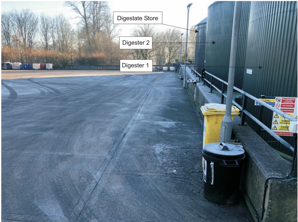
Photo 5. Retaining bund (wall) along northern margin of site
