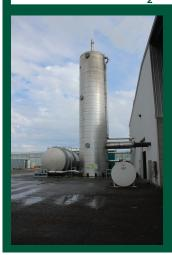
The alternative to selectively removing the pollutants is to extract the CO<sub>2</sub> directly. The most common method is to use an amine scrubber. This was the principle introduced in a Canadian system, developed in late 2013 (ProCeed), and which has subsequently been adopted by a small number of companies in the UK and Europe.
