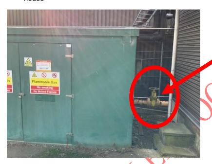
Turn the valve clockwise to shut off the gas supply to Bruton Site.
