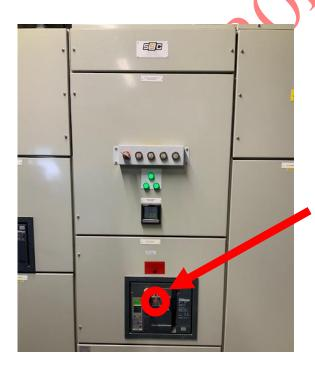
Lift the plastic screen and push the red button to shut off the electric to Bruton Site.
