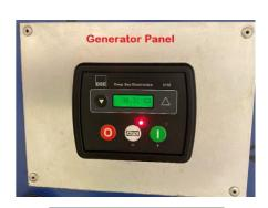
Turn off the back up generator otherwise this will start when the electric is shut off.
