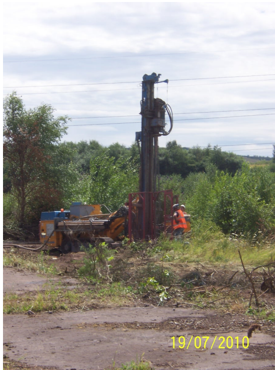
Photograph 11: Investigation undertaken by Hydrock to determine locations of mine shafts
