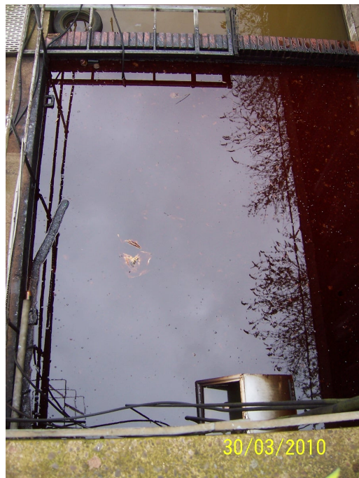
Photograph 20: Evidence of hydrocarbons on surface of water in interceptor tanks
