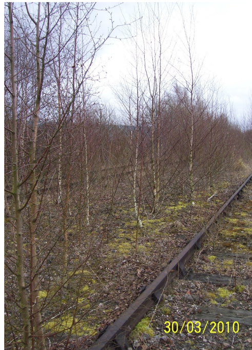
Photograph 7: Railway sidings located on the north edge of the site
