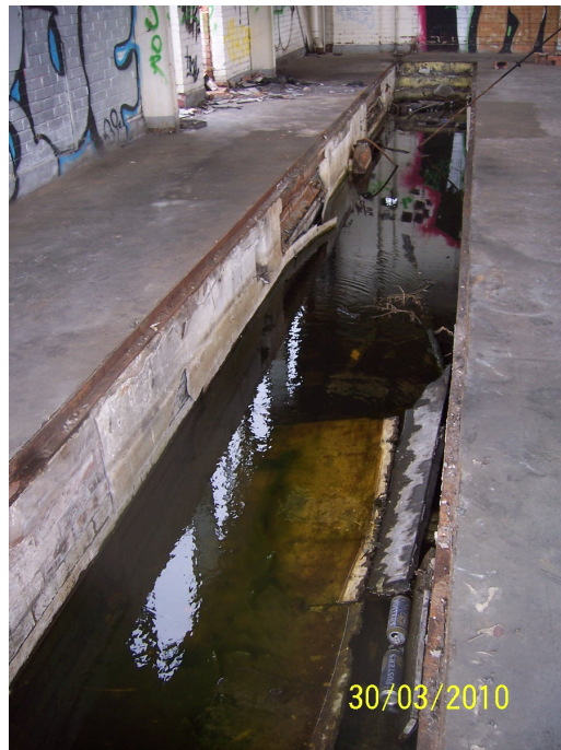
Photograph 9: One of the inspection pits located inside the workshop buildings
