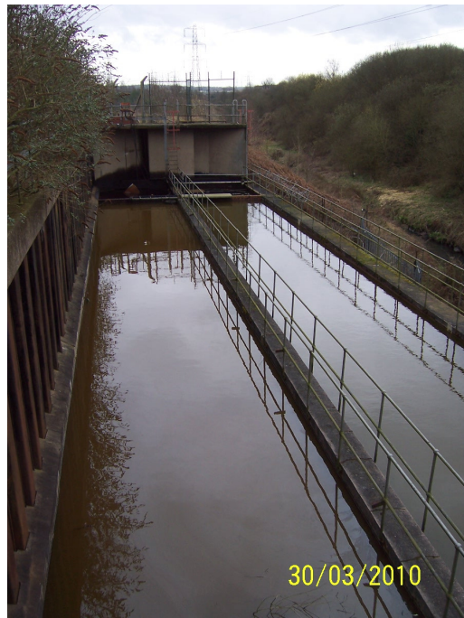
Photograph 19: Old Interceptor tanks looking south
