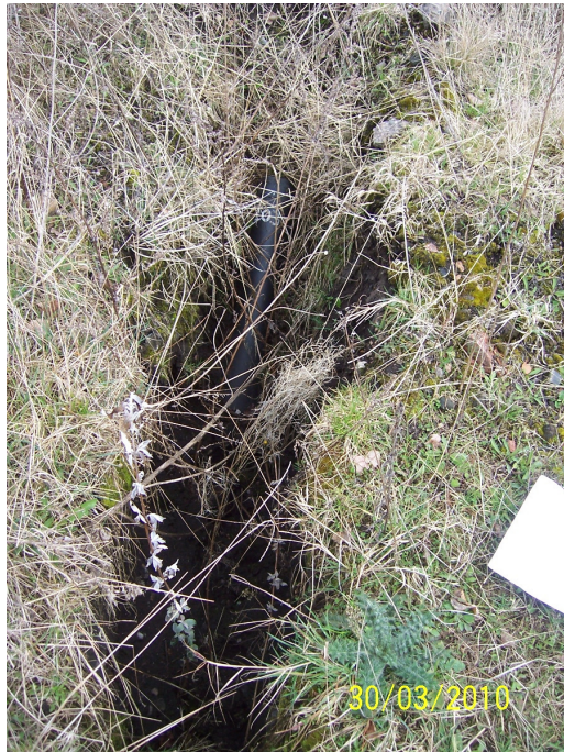
Photograph 21: One of the ruined boreholes
