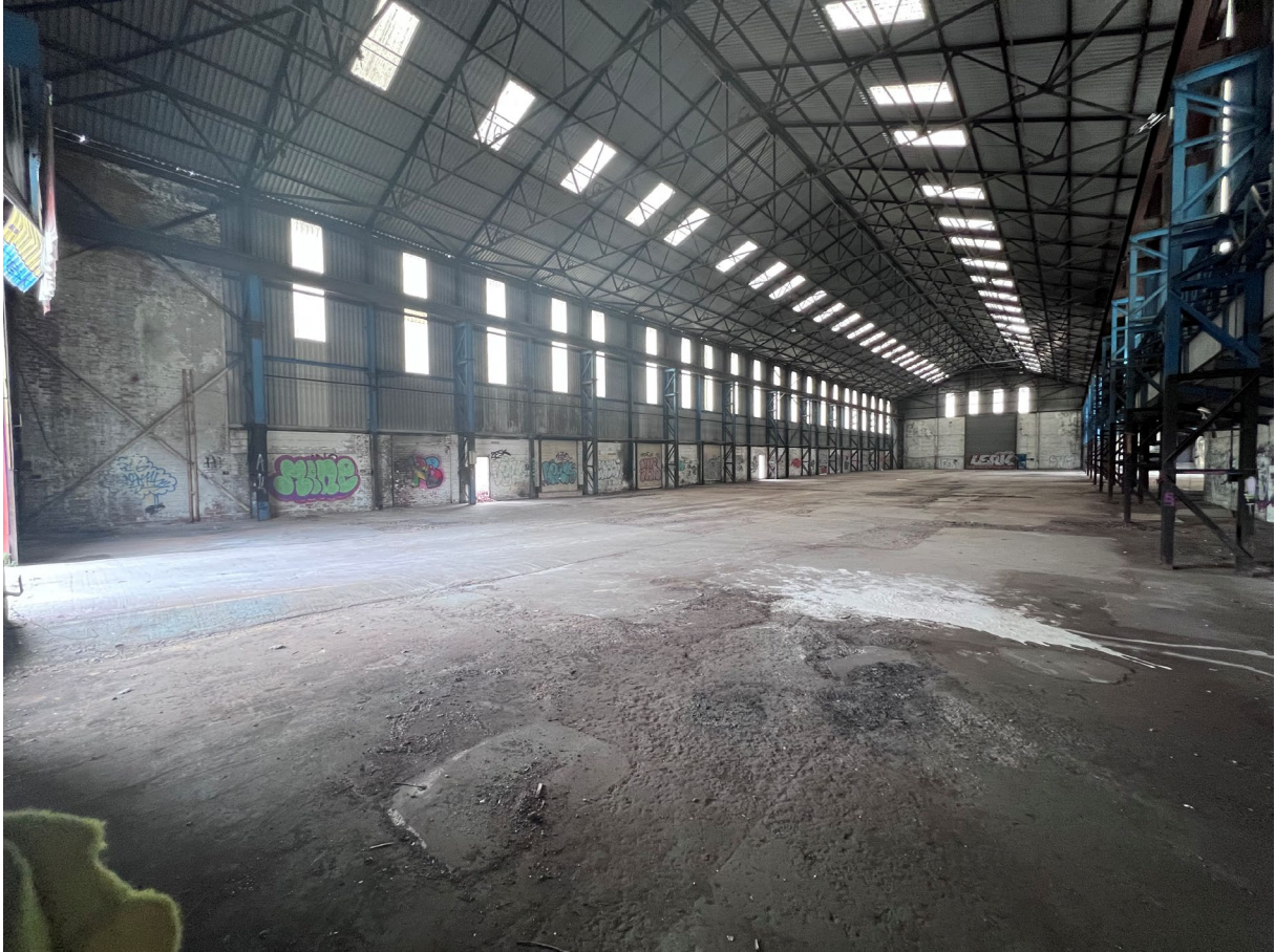
Photograph 6 Inside main building, looking north east
