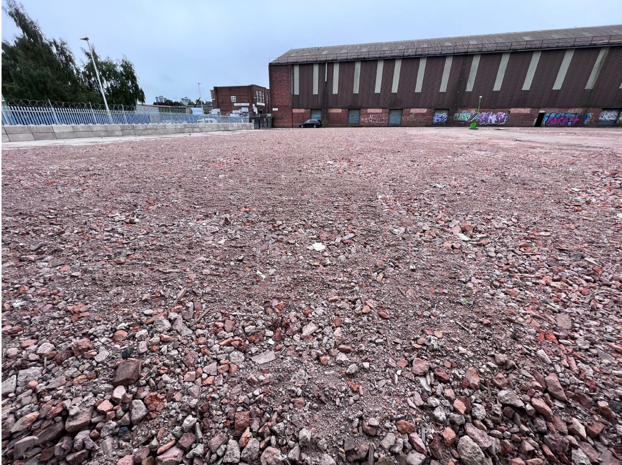
Photograph 2 View south across north eastern area of site
