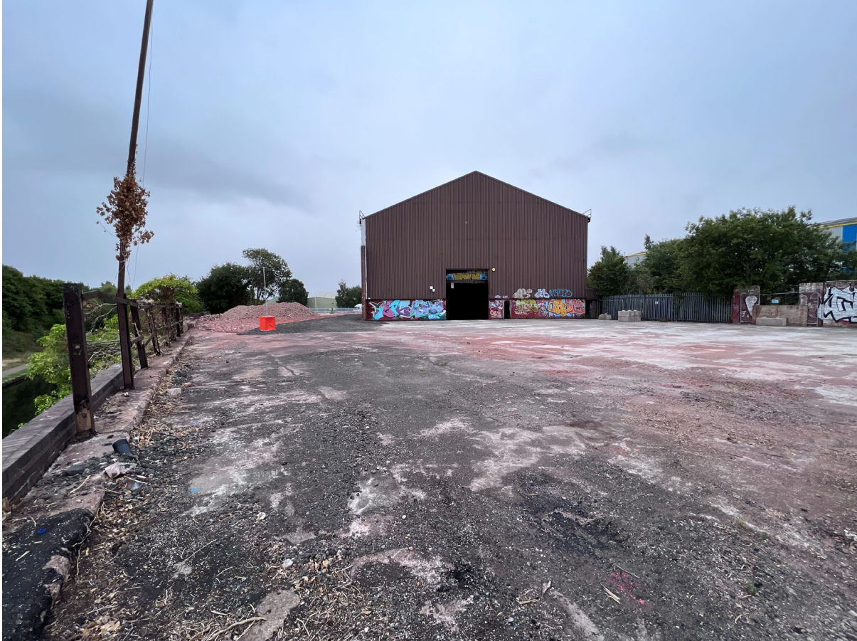
Photograph 3 Main building on site viewed from west
