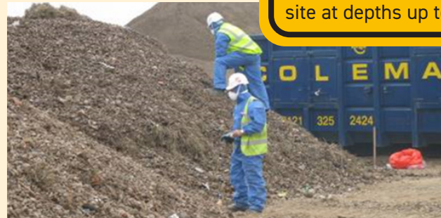
Asbestos finds—hand picking | Ramboll
