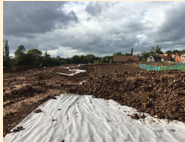
Installation of the cover system | AECOM
