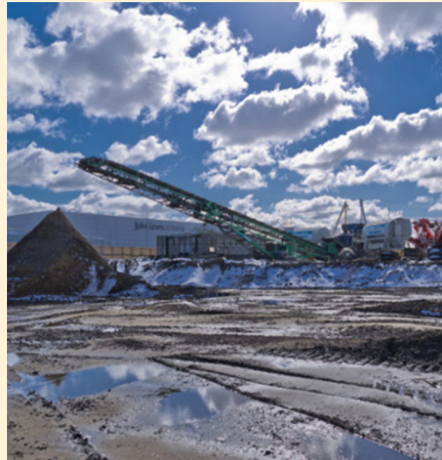
Processing plant | John F Hunt
