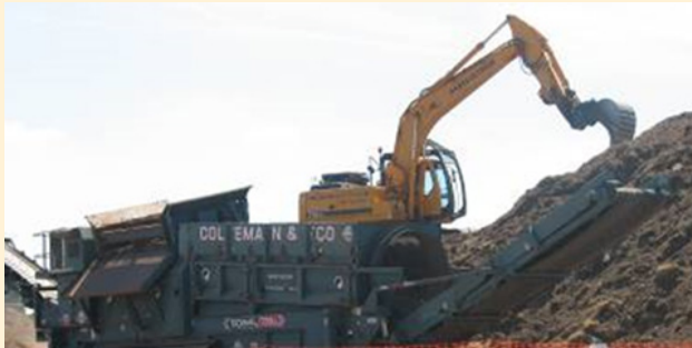
Processing plant | Ramboll
