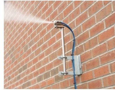
Figure 13 : Unit 2 spray nozzle
