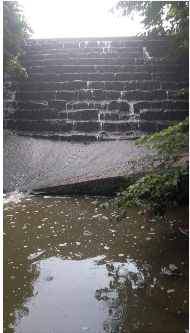
Figure 2: Overspill dam weir from above and below.
