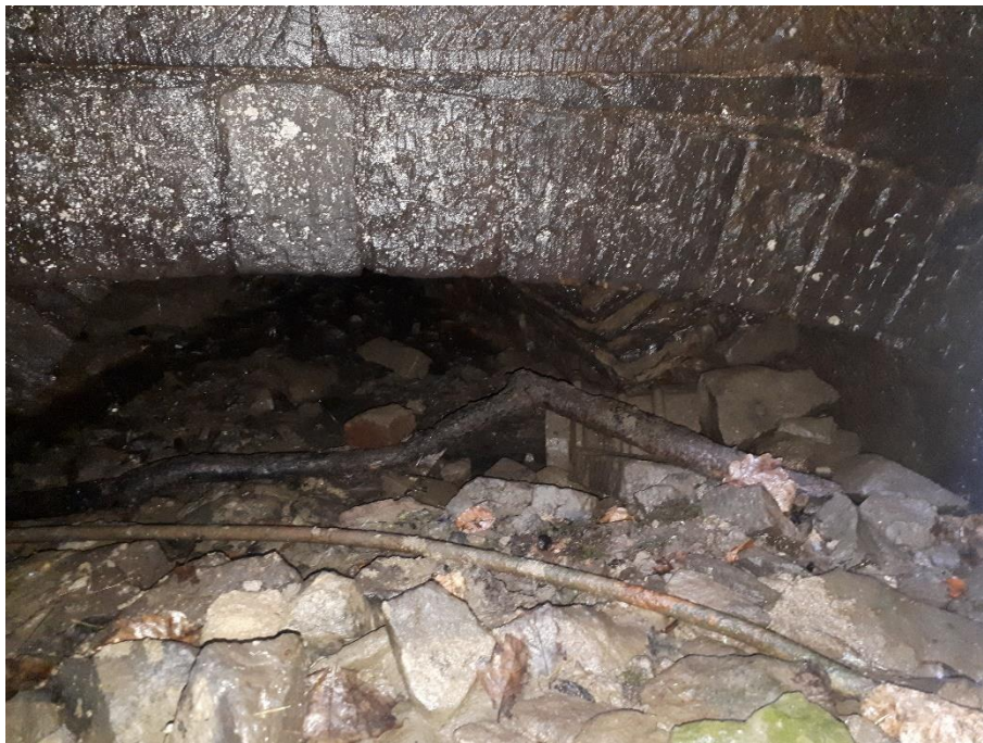
Figure 5: entrance to the culvert in the wheelhouse.
