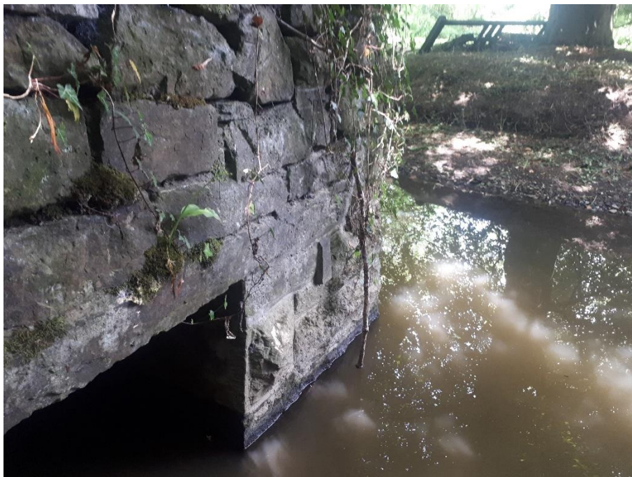
Figure 7: view looking across The Moss from the culvert discharge.
