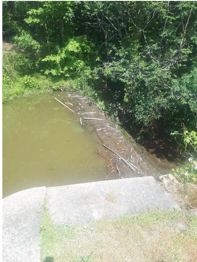
Figure 1: view looking across the existing weir.
