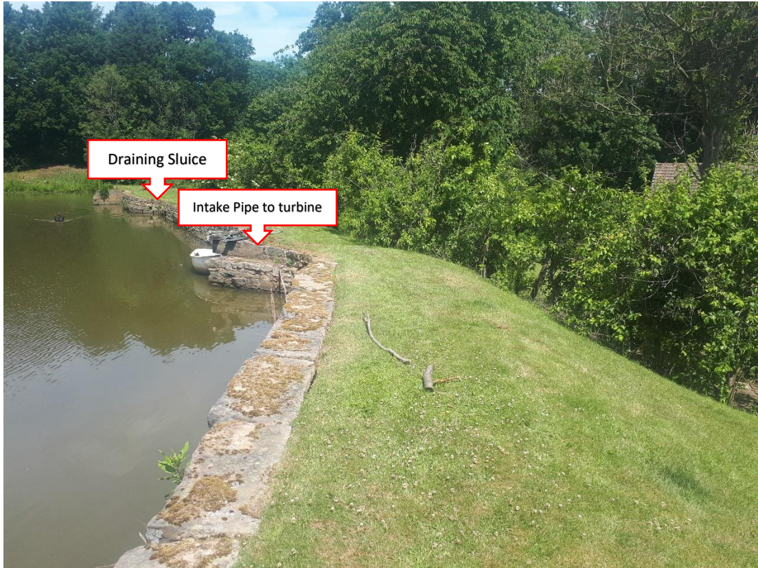
Figure 3: Mill Pond draining sluice and intake pipe to turbine house location
