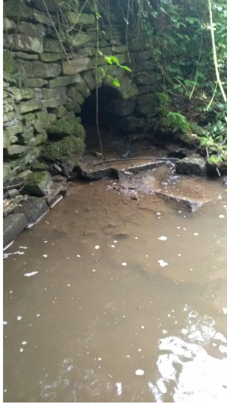
Figure 5: Tributary culvert outfall, 85m downstream of weir.
