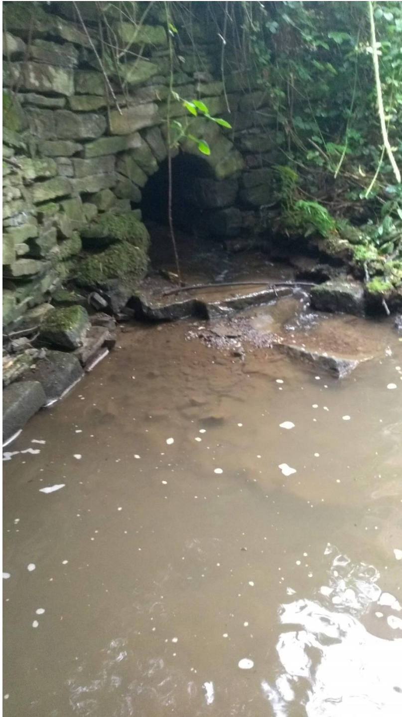
Culvert outfall of tributary to the Moss shown in figure 1.
