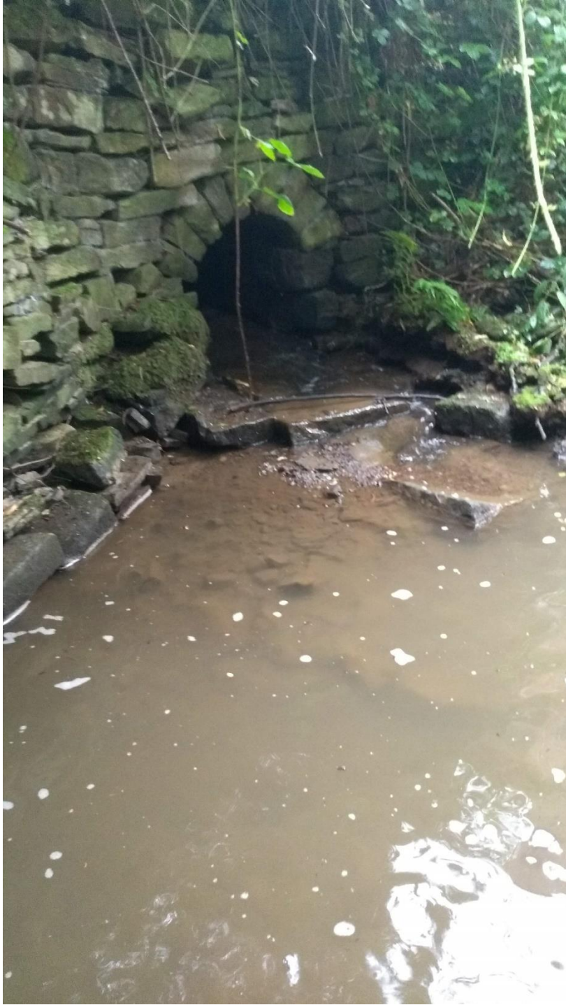
Culvert outfall of tributary to the Moss shown in figure 1.
