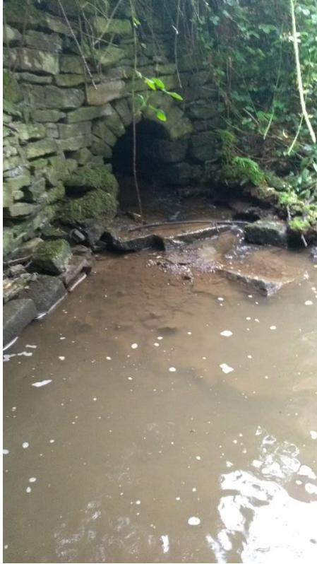
Figure 5: Tributary culvert outfall, 85m downstream of weir.
