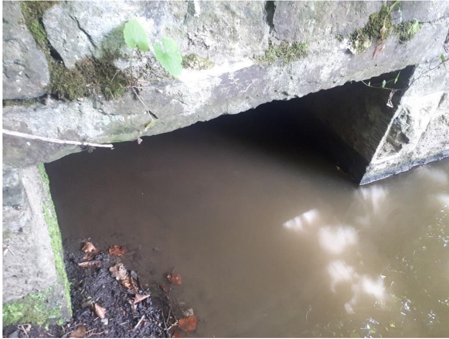
Figure 6: discharge from the culvert to The Moss.
