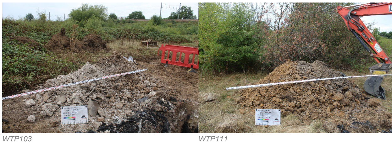
Figure 3: Example of Made Ground Encountered
