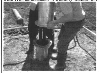
Northerly CMT well at PNR awaiting gas clam and headwork's fitting:
