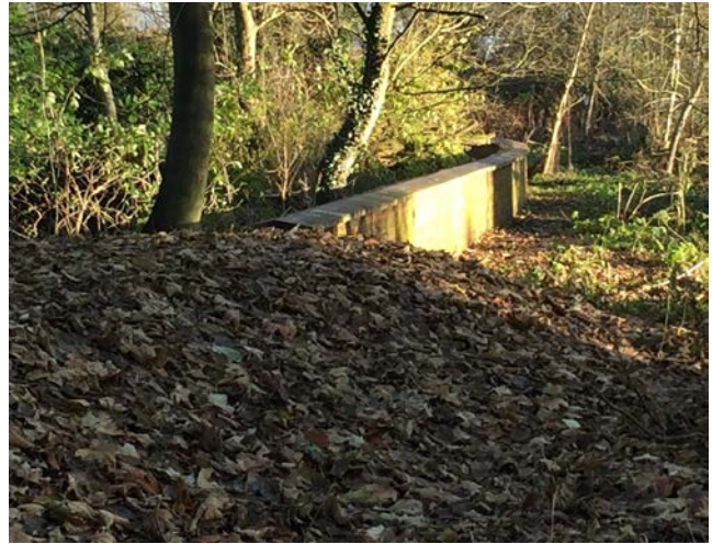
Earth embankment and wall on the right bank, near the Memorial Hall car park.)
