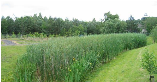
Reed beds at the Acomb coal mine water treatment scheme
