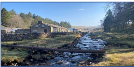
The existing pipe bridge near Nenthead car park
