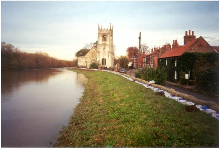
Photo: Sandbags on top of the flood defences in the village of Cawood to prevent 'overtopping'.
