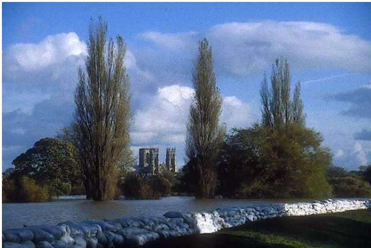
Photo: Sandbags on the downstream end of Clifton Ings at Water End stopping excess water from flowing through York.
