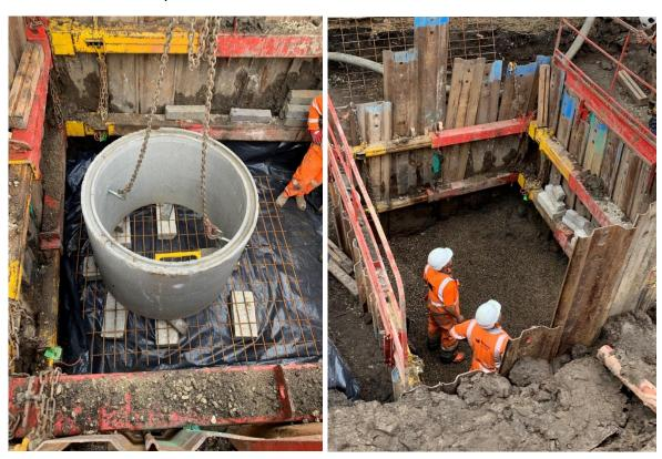
Photos showing the installation of base concrete and pipework during the manhole relocation works Following this, works on the embankment will resume, and are on track to be completed in the New Year.
