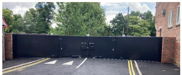
Fig. 2 New Flood Gate at Clementhorpe Junction
