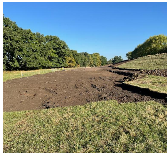
Fig. 4 Site with MG4 grassland safely cut and lifted out
