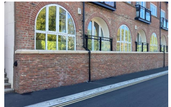
Fig. 1 New Flood Wall at Waterfront House
