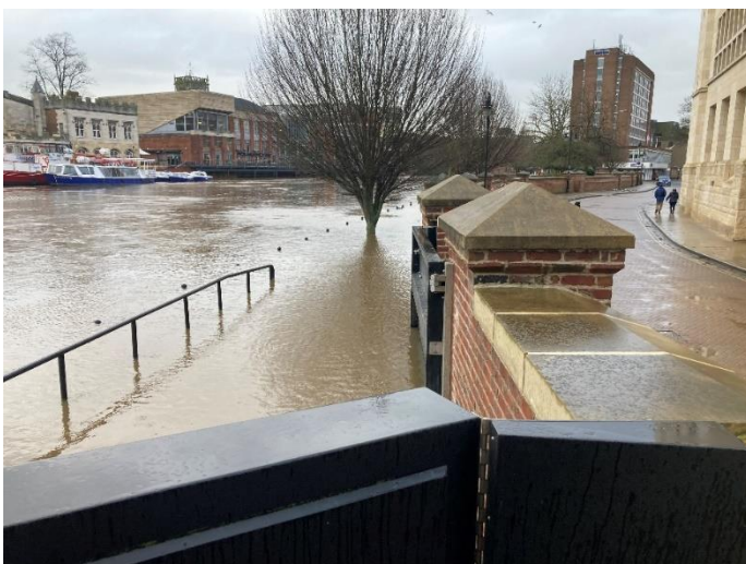
Our North Street defences in action during the February 2022 flooding in York
