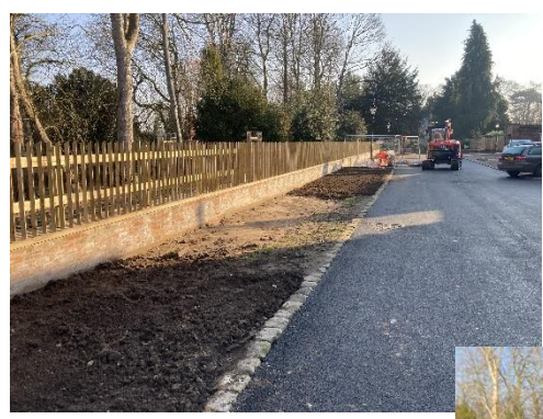
Completed underground defences and flood wall
