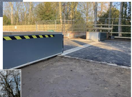
Completed flood gate at the end of Chantry Lane
