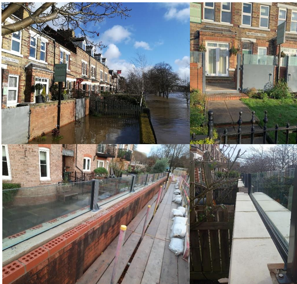
Top left: Flooding by Earlsborough Terrace February 2020. Bottom left: Installing the new flood panels December 2021. Top and bottom right: Completed flood panel installation
