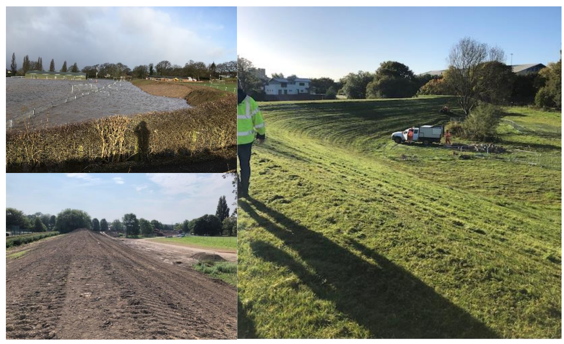
(Top Left: St Peter's School sports fields flooded February 2020. Bottom Left: Construction work taking place to increase height of the Lower Bootham embankment August 2020. Right: Works to raise the height of the embankment complete)
