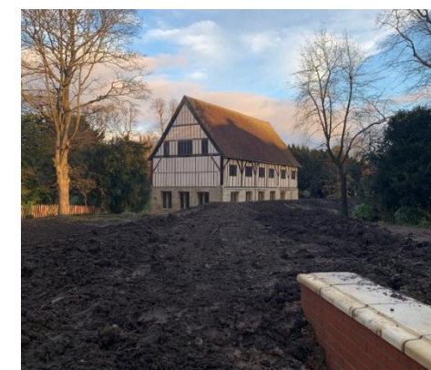
Work on the Museum Gardens embankment December 2021
