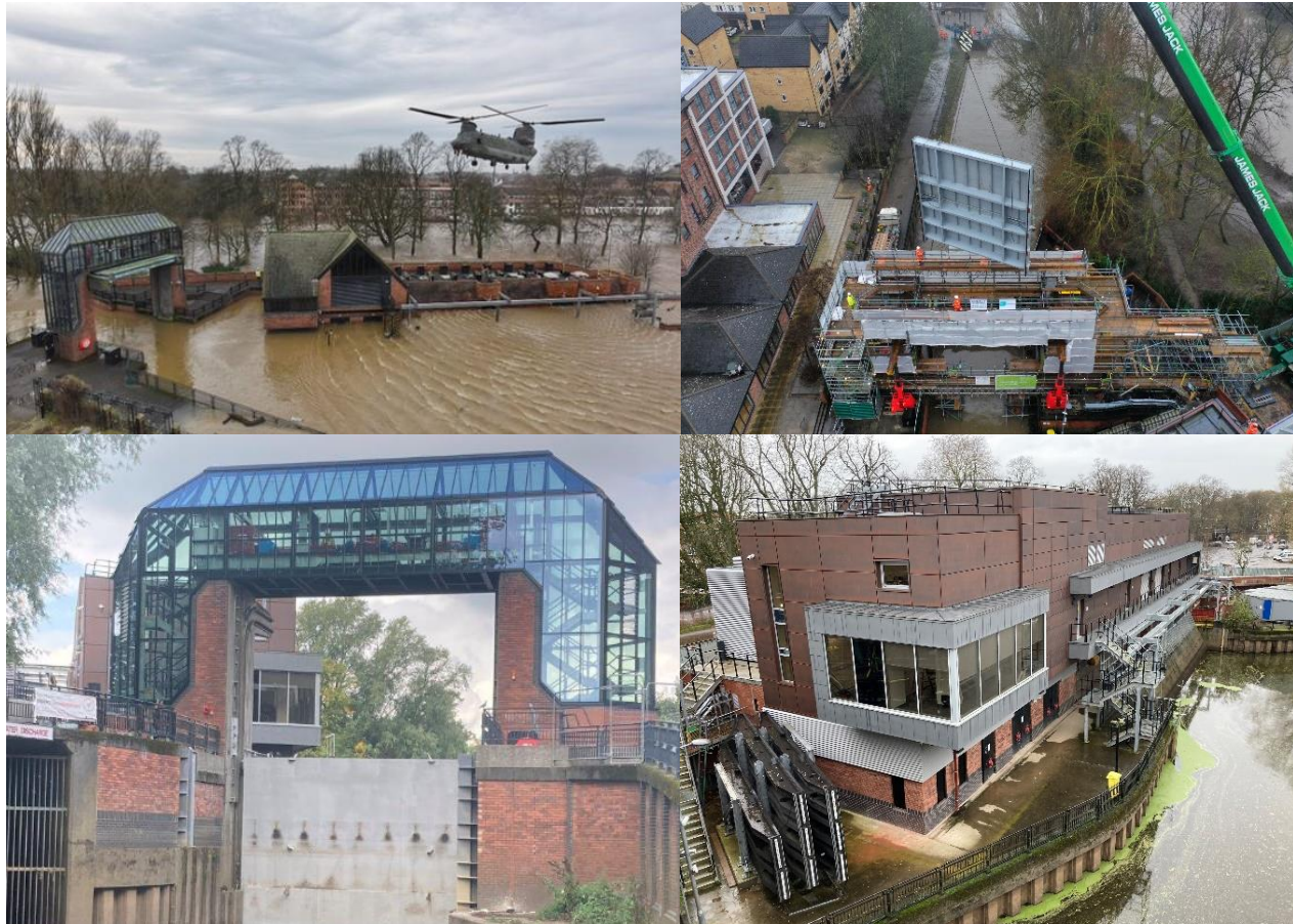
(Top Left: Foss Barrier during the Boxing Day 2015 flood event. Top Right: The new gate installation January 2021. Bottom Left and Right: Newly upgraded Foss Barrier)
