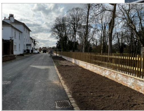
Completed flood along Chantry Lane
