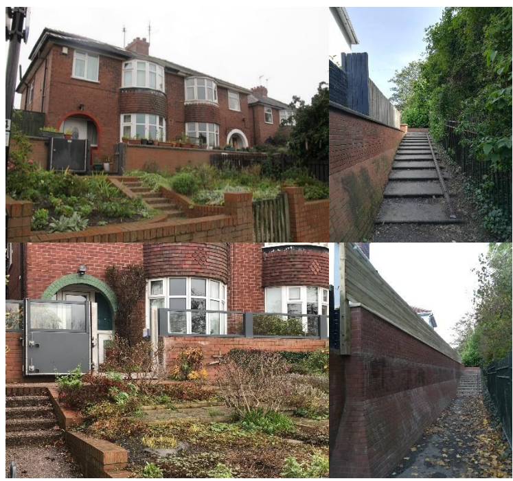
(Top Left: Almerly Terrace properties prior to our works. Top Right: Almerly Steps flood wall prior to works. Bottom Left: New glass panels on Almerly Terrace. Bottom Right: Newly raised Almerly Steps flood wall )
