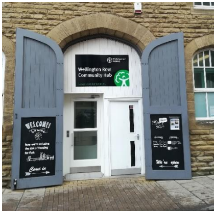
York Community Flood Hub entrance, Wellington Street
