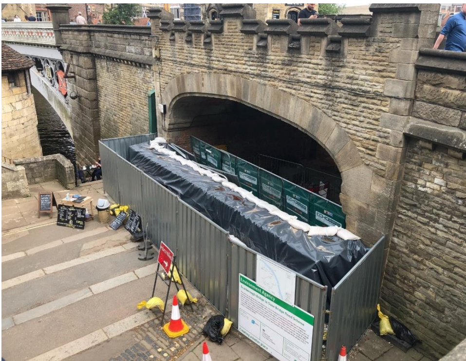
Figure 1 - Work continuing installing our new and bigger flood gates under Lendal Arch on 23 June 2021
