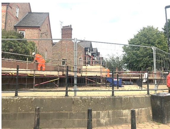
Figure 3 – Photo of works being done to raise the flood wall from Scarborough Bridge to Marygate on 23 June
