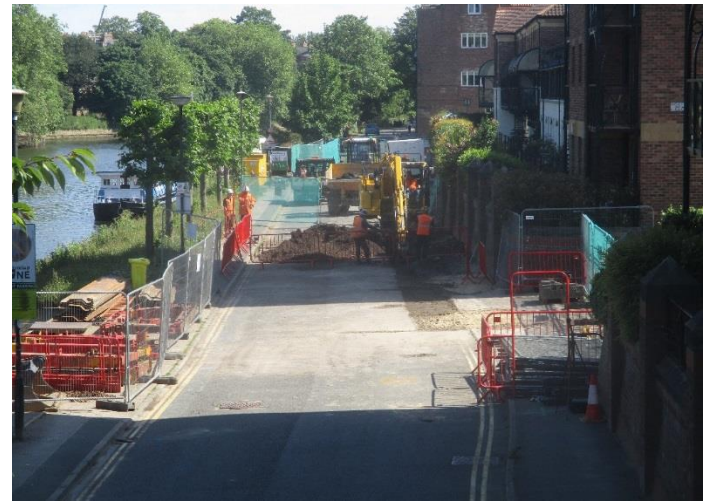
Figure 2 - A picture of the work being done on Terry Avenue on 22 June 2021
