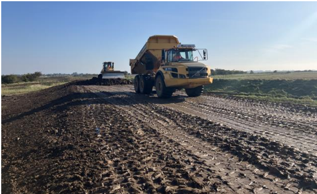
Photo 2: A dumper and dozer moving and laying material on the embankment
