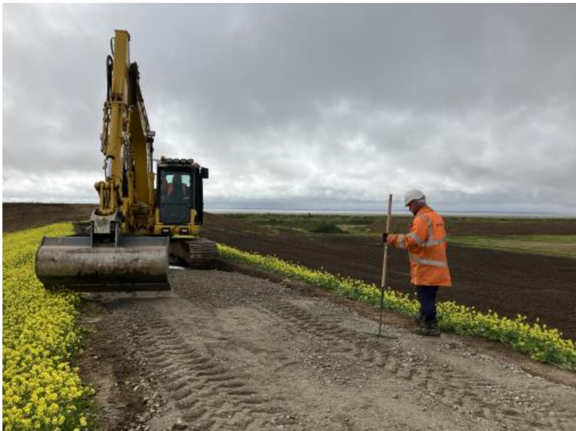
Photo 3: building the path on top of the new embankment
