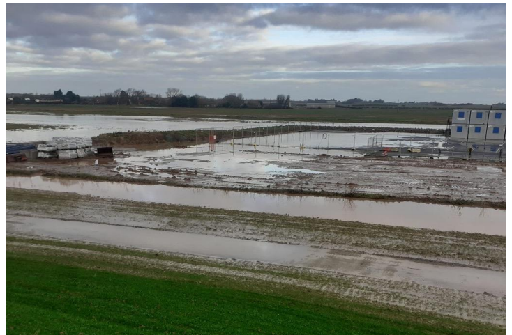
Photo: View of the Weeton site compound, January 2024.
