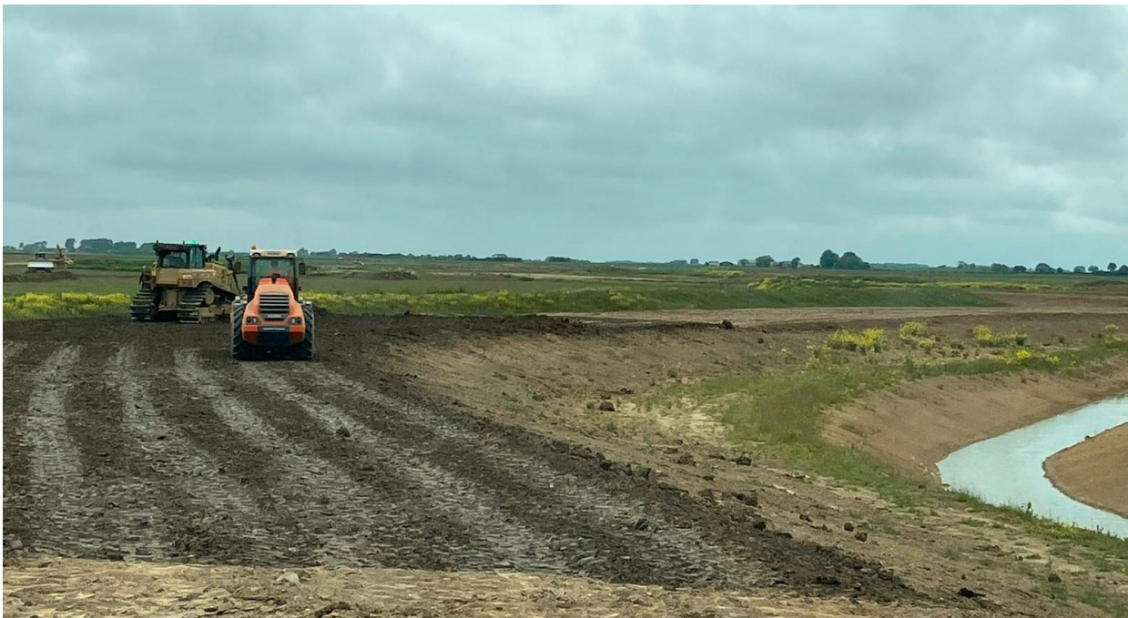
Photo showing machinery placing and compacting the clay core for the new flood embankment
