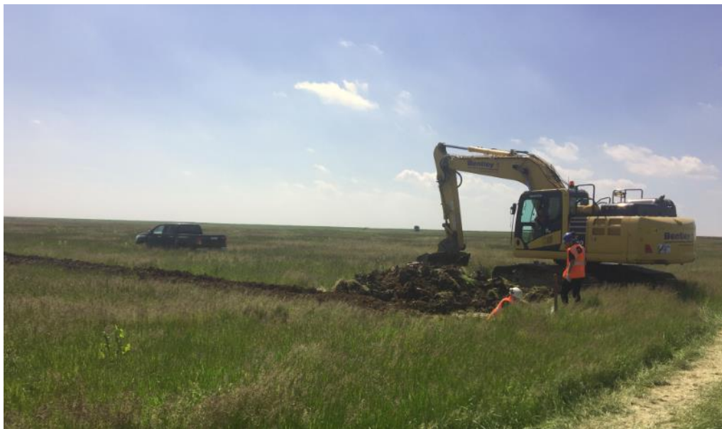
A pit being dug for geotechnical surveys on site
