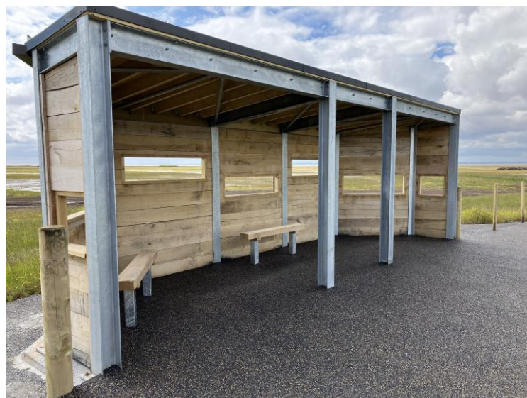
One of the new bird hides recently installed, with Flexipave surfacing in place.
