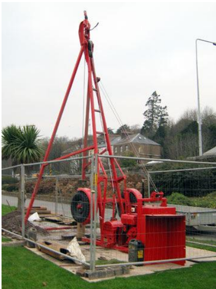
A construction rig for digging boreholes for ground investigations
