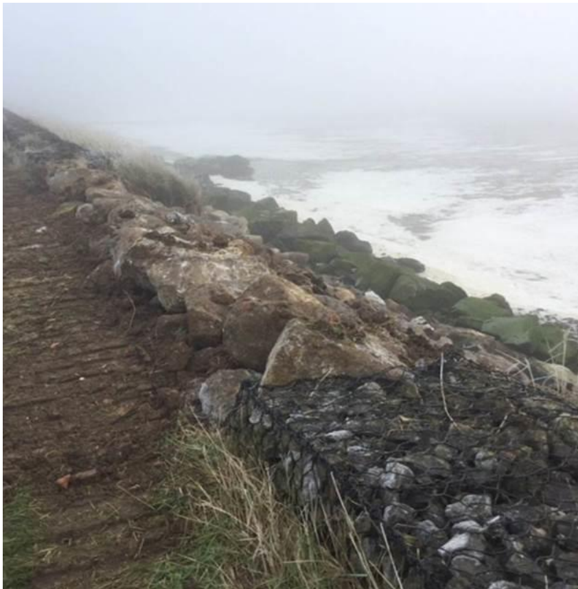
The repaired embankment below Outstrays Farm with new gabions in place.
