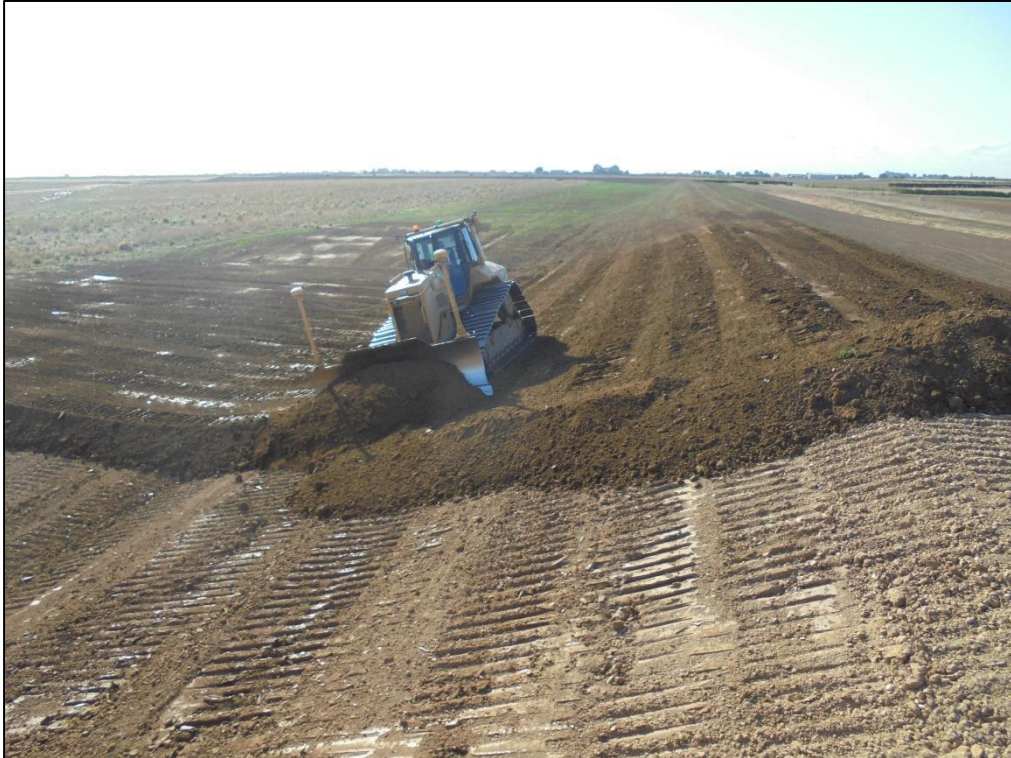
Photo: Trimming and topsoiling of the new flood embankment
