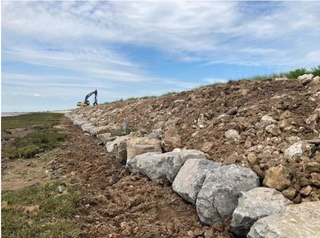
*Repairs being made to the embankment between Skeffling and Easington*
