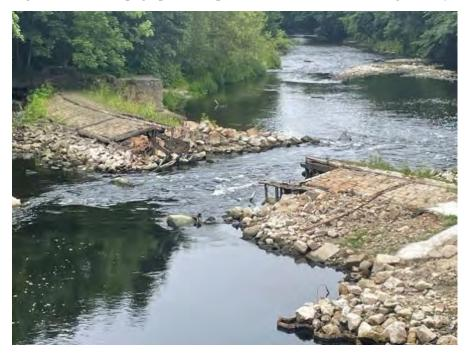
Figure 35 Breached Weir (June 2021)
