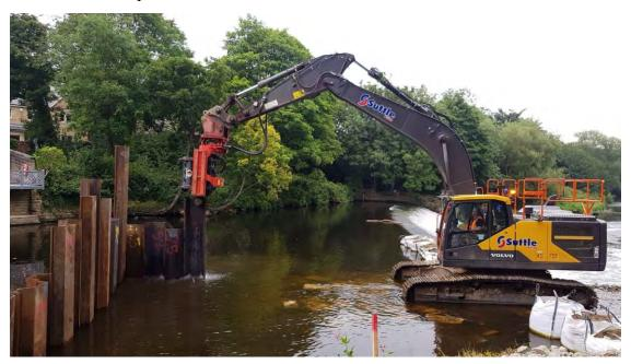
Figure 17 Piling installation for cofferdam
