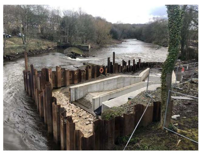
Figure 5 : Photograph showing the collapsed weir during construction of the fish pass.
