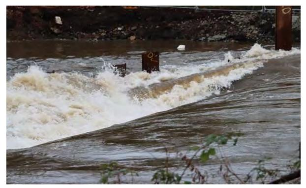
Figure 44 Turbulence and flow deflection across face of the weir – 21st Jan 2021
