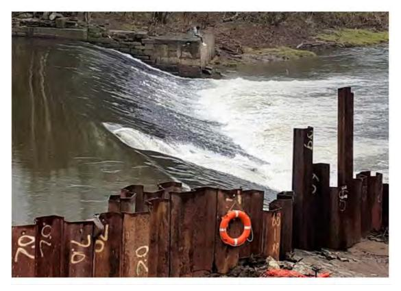
Figure 54 Initial weir failure (21-01-2021)
