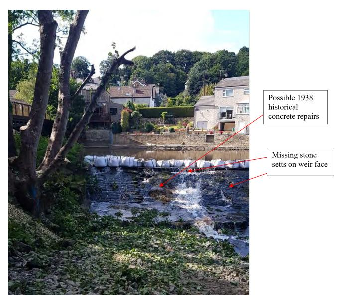
Figure 14 Sand bags placed on weir to allow access (taken by the Environment Agency)
