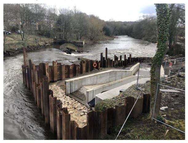
Figure 26 The collapsed weir during construction of the fish pass
