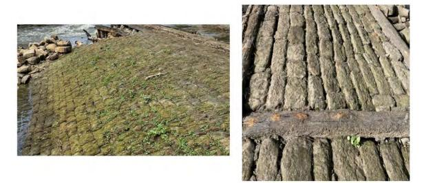
Figure 7 Build-up of the stone blocks on downstream and upstream face on Newlay Weir (11-05-2021)
