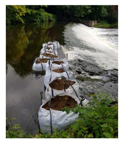
Figure 13 Sand filled bags to allow access to the weir (taken by the Environment Agency)
