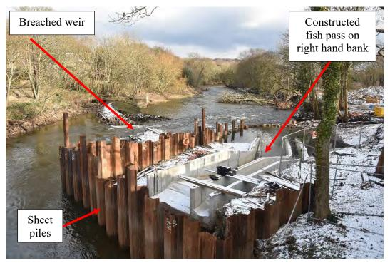
Figure 1 Newlay Weir post failure (12-02-2021)
