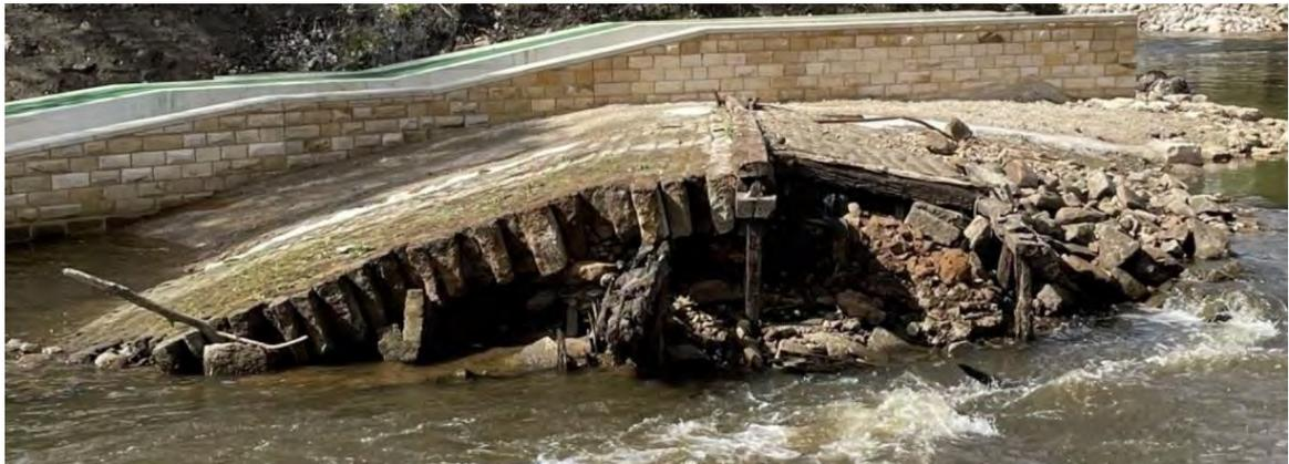
Figure 5 Construction/build-up of Newlay Weir (11-05-2021)
