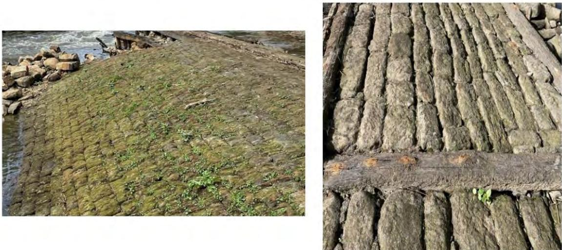
Figure 7 Build-up of the stone blocks on downstream and upstream face on Newlay Weir (11-05-2021)
