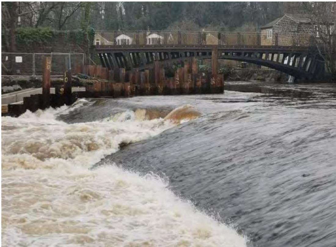
Figure 58 Progression of front face failure (04-02-2021)
