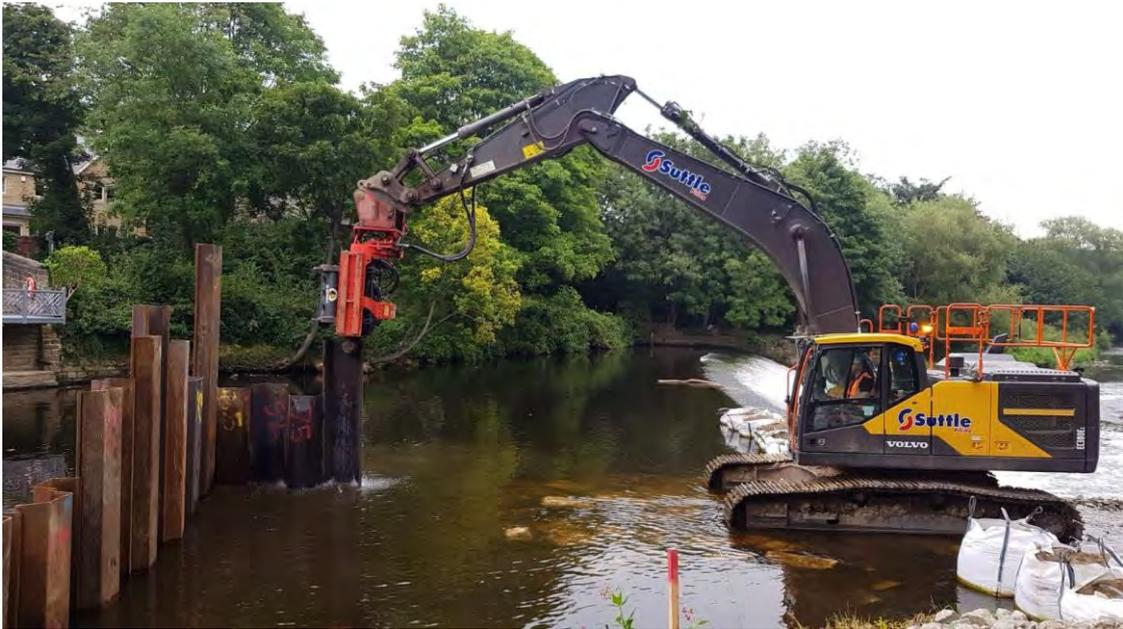
Figure 17 Piling installation for cofferdam
