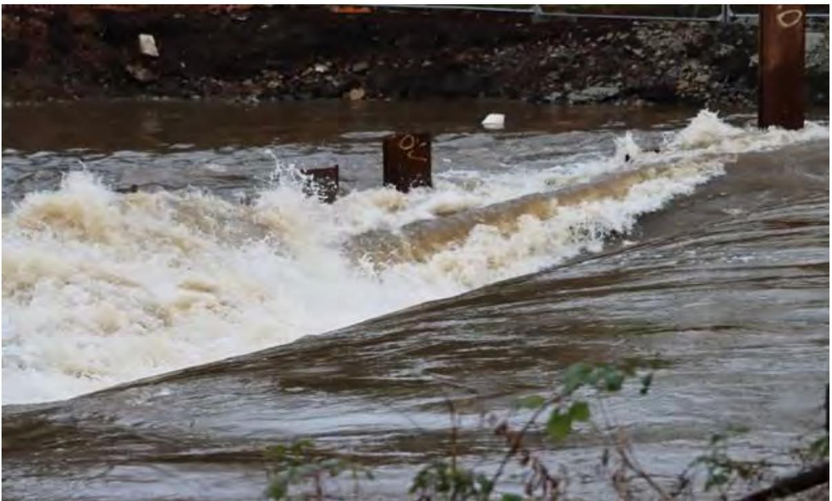
Figure 44 Turbulence and flow deflection across face of the weir – 21<sup>st</sup> Jan 2021
