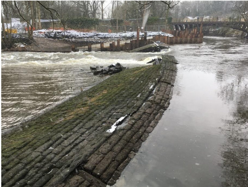
Image showing collapsed section of weir.
