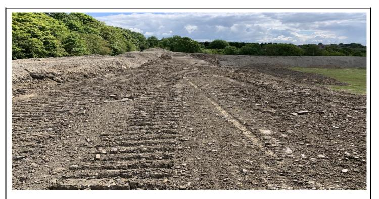
Advised John to continue with visual inspection of material being used and remove any oversize or clods that are observed and condition (i.e. add water) to aid compaction if soils become too dry. Any oversize material removed from the load is being stockpiled on site for use on haul road as the site develops or discarded over the inner flank of the bund.
