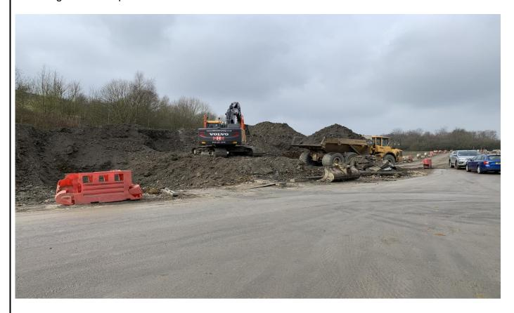
Any oversize material removed from the load is being stockpiled on site for use on haul road as the site develops.
